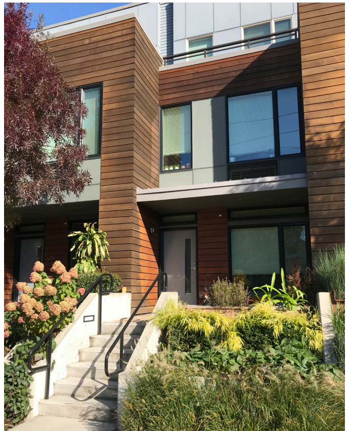
Bays create upper-level decks and provide recesses for entries while differentiating units from one another.
