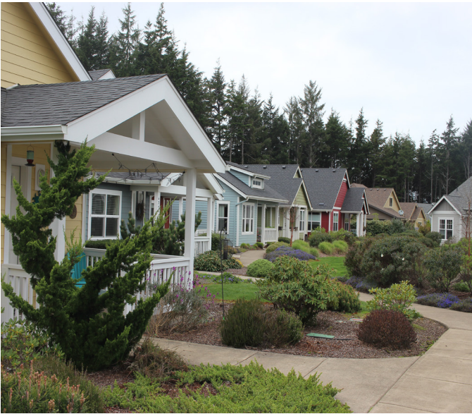
Cottage on the corner has setback from the walking path.
