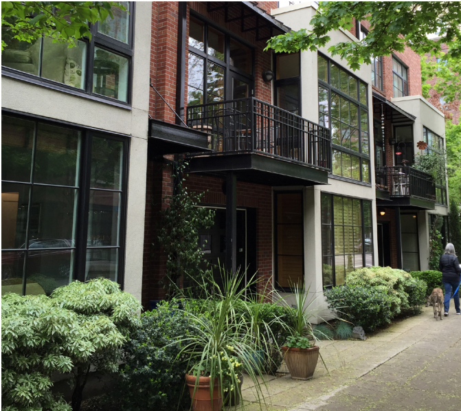
Gateway zone is created by projecting bays on either side of the entry, while a balcony above provides rain protection on the ground level.
