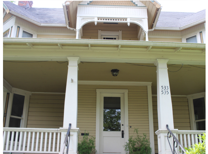
Single dwelling converted into a duplex.
