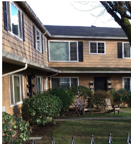
2-story courtyard apartment
