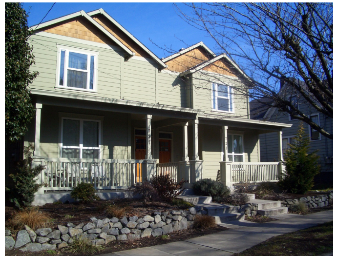
A porch railing separates entries and provides privacy to each unit, while creating a cohesive porch across the front.
