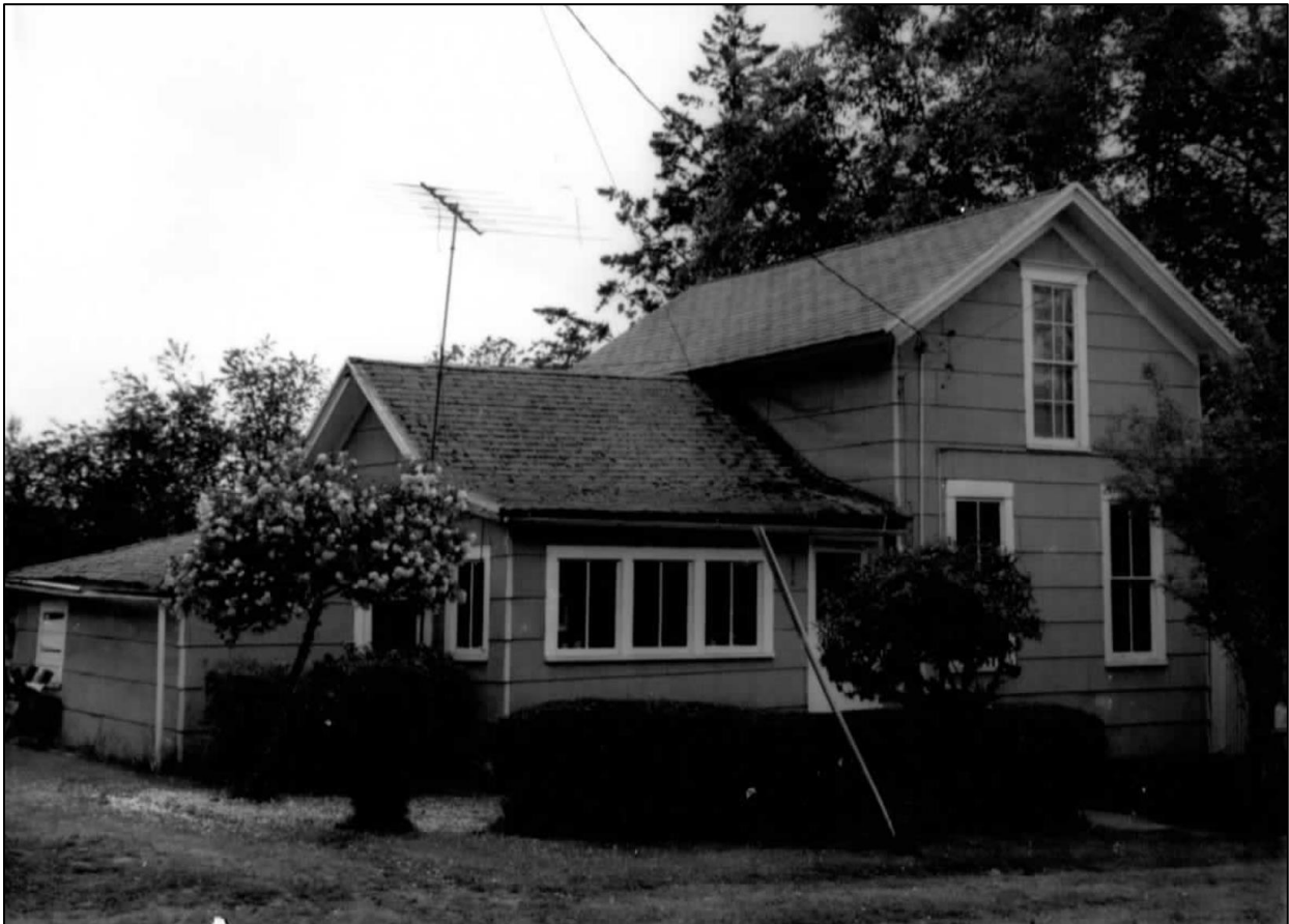
Figure 2. 1983 Historic Resources Inventory Photo
