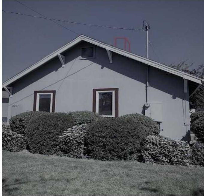
Image 2 Existing Street Elevation 423 College depicting removed chimney
