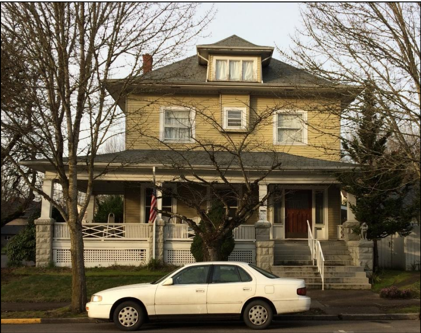
605 NE 1 st Street
