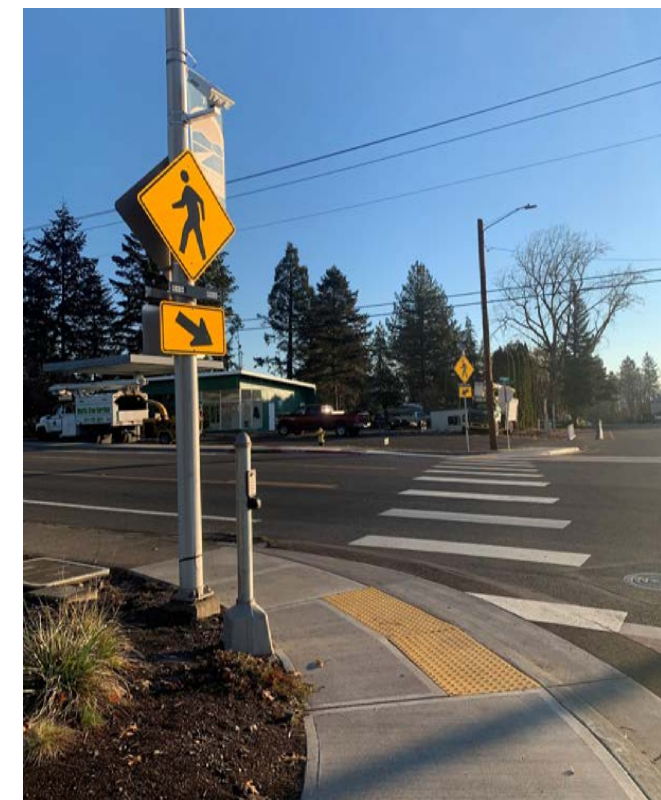
Rectangular Rapid Flashing Beacon
