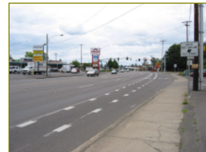
Bike Lane on Highway 99W
