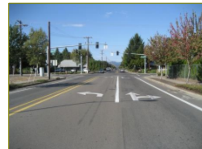
Bike Lane on Baker Creek Rd
