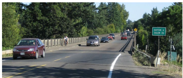
Limited Sidewalk Width on Yamhill River Bridge
