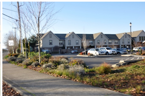
Central Neighborhood and CCC Area
