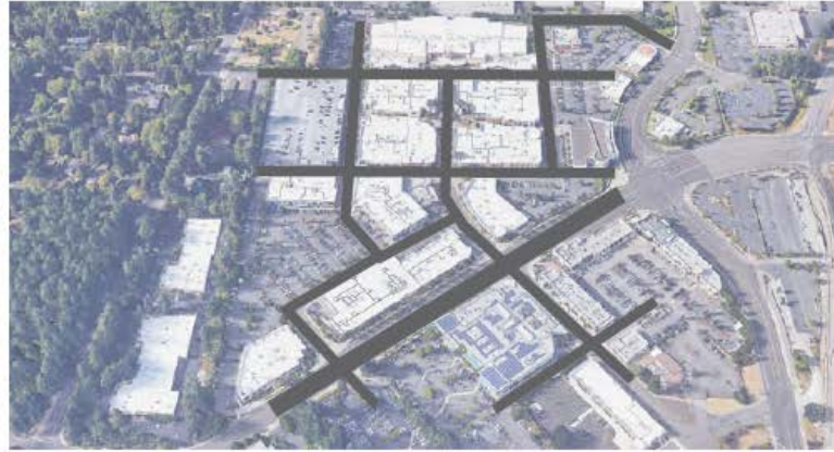
Establish connected blocks on grid of internal circulation (Bridgeport Village example shown)
