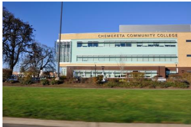
Central Neighborhood and CCC Area
