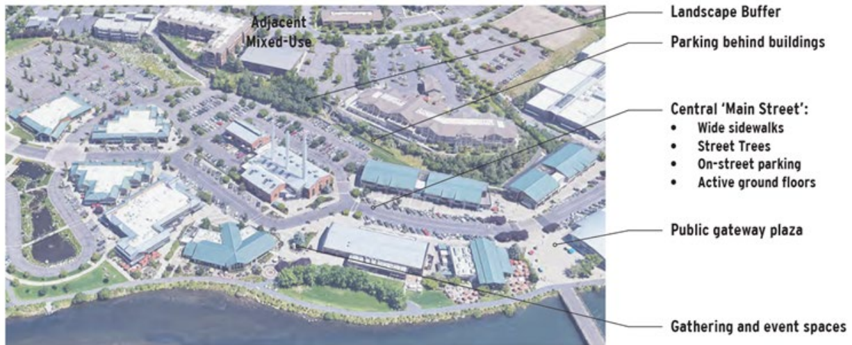
Figure 3. Retail Center Precedent: Old Mill District, Bend, Oregon
