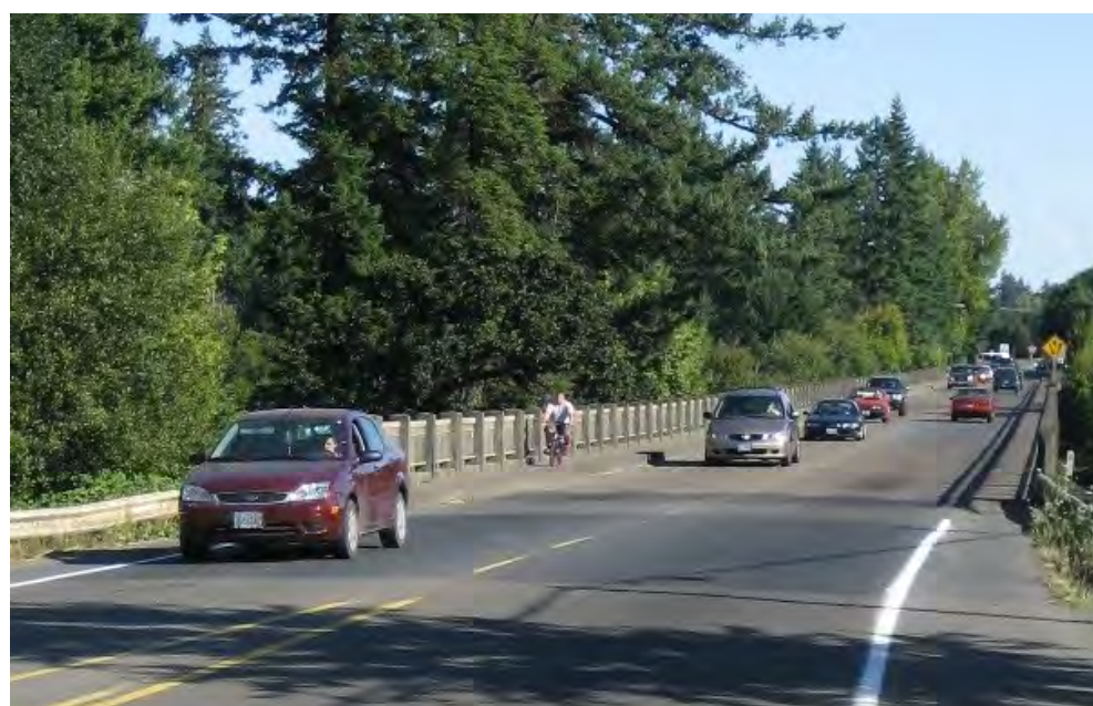
Narrow sidewalk, no bike lanes on Yamhill River Bridge
