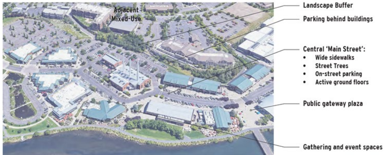
Figure 9. Retail Center Precedent: Old Mill District, Bend, Oregon
