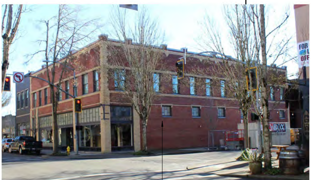
2 STORY (35' HEIGHT) BUILDING SOUTH OF PROPERTY
