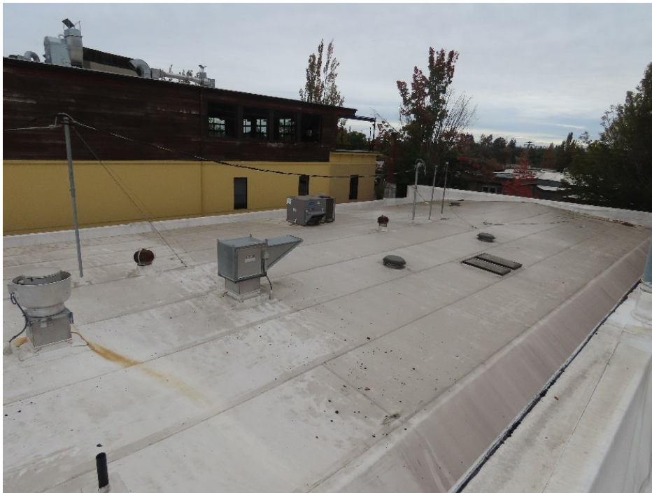
Photo 24. Roof overall view looking south (ARG, October 2022).
