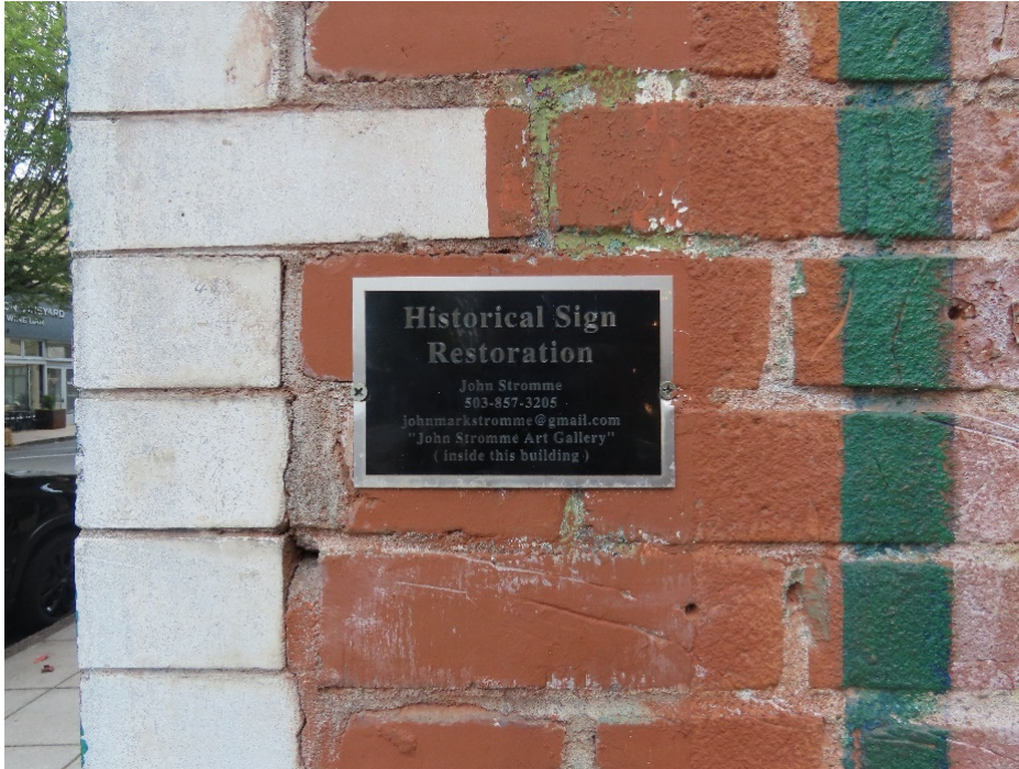
Photo 23. East elevation detail at southeast corner, unpainted white face brick at left (ARG, October 2022).
