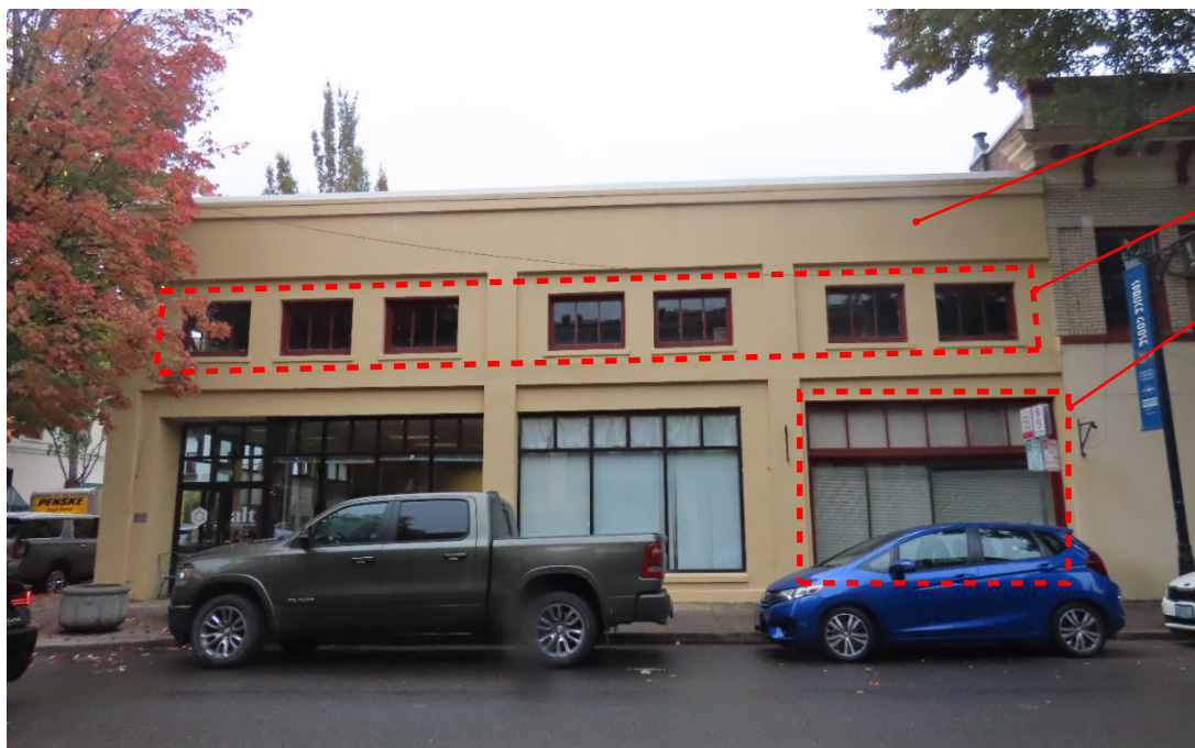
South Elevation facing NE Third Street, illustrating original features (ARG, October 2022).
