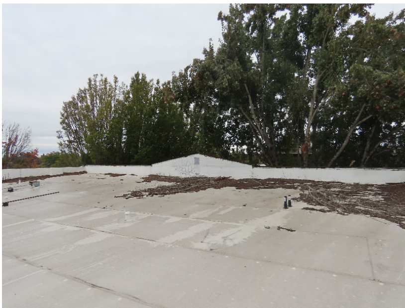
Photo 16. Roof looking south (ARG, October 2022).
