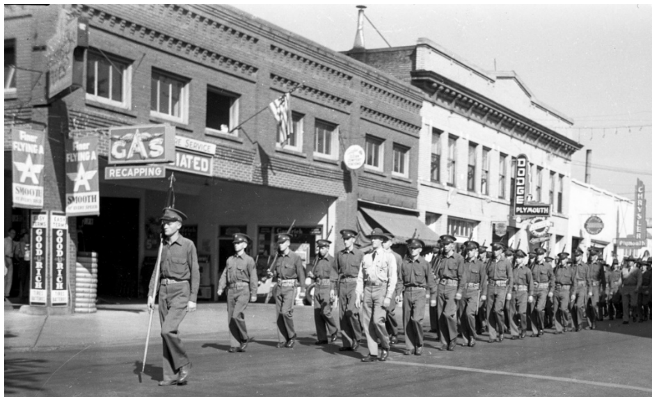
The ground floor was reconfigured to accommodate gasoline pumps prior to this 1940 photograph (Yamhill County News-Register).
