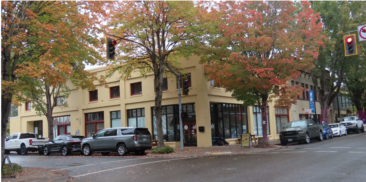
The bays at the corner of the ground floor have been infilled with the current street-facing storefront; three original storefront bays remain (ARG, October 2022).
