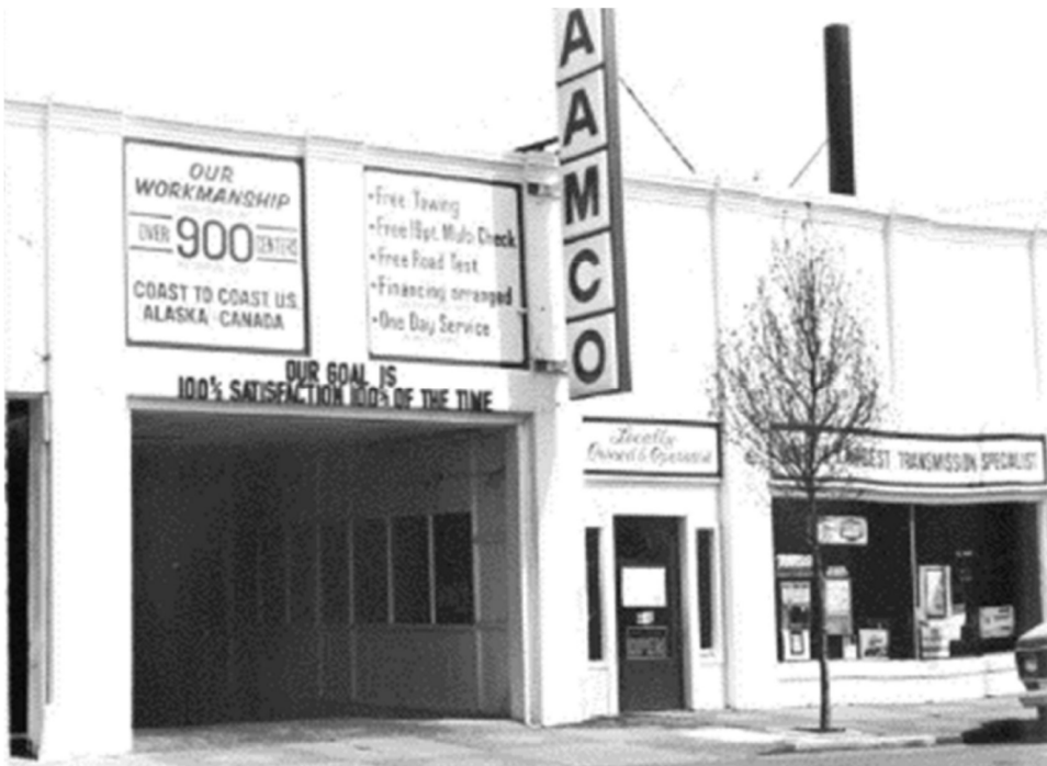
By the time of this 1983 historic survey photograph, the window to the east of the double-wide opening had been converted to an entry and the windows in the two easternmost bays had been replaced with a storefront window spanning both bays (Historic Resources Survey, City of McMinnville, Yamhill County, Oregon).
