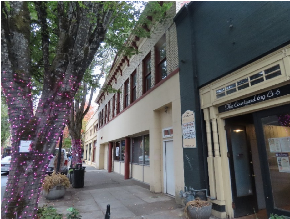
Photo 9. Overall view of south elevation, showing modified ground floor and original second floor (ARG, October 2022).
