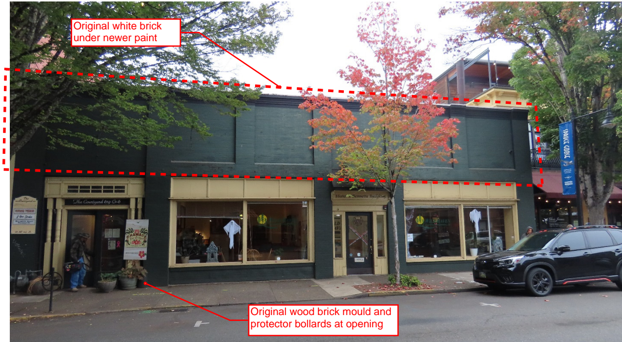
Current view of 619 NE 3rd Street (ARG, October 2022). Paired doors with wood trim elements have been inserted into the westernmost bay, while the formerly double-wide opening has been replaced with a storefront window matching the window in the easternmost bays.
