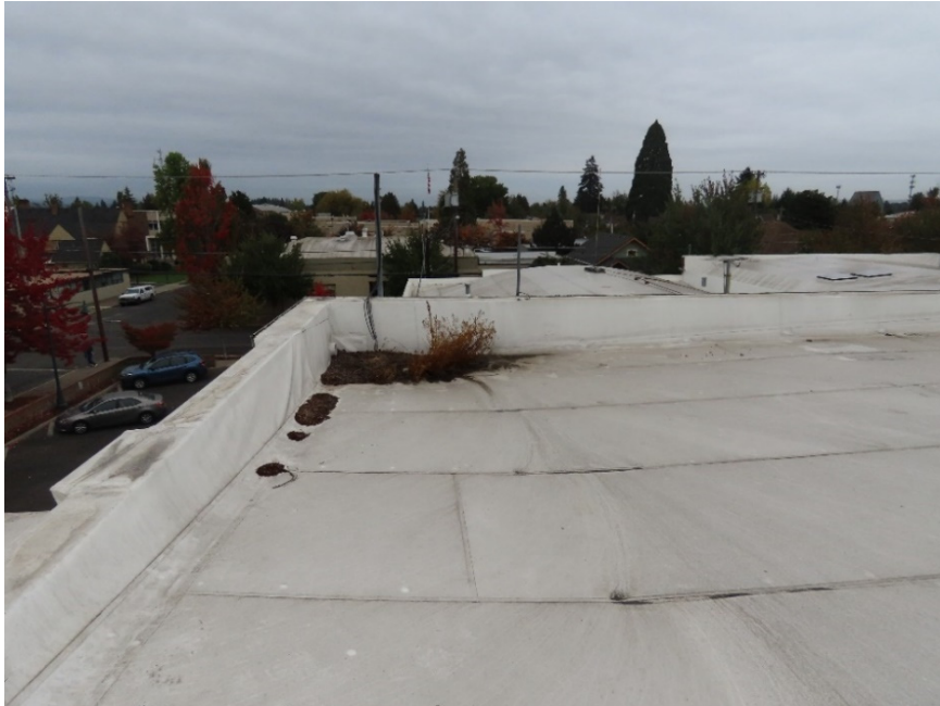
Photo 17. Roof looking north; note debris at location of roof drain (ARG, October 2022).
