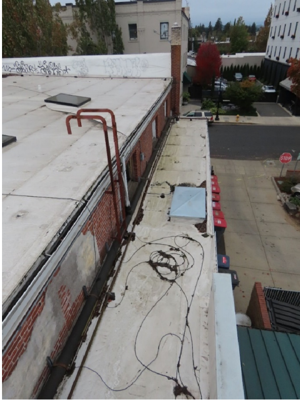
Photo 5. Replacement roofing; main roof at left, one-story north bay at right (ARG, October 2022).
