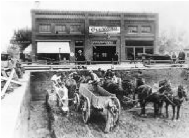
A c. 1904 photo from soon after 609 NE 3rd Street’s construction, showing the brick exterior and original ground floor configuration (Yamhill County Historical Society).
