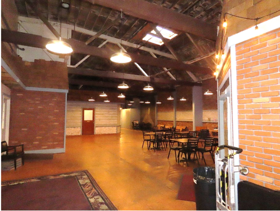
Photo 25. Interior view with wood trusses above (ARG, October 2022).
