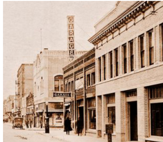
A 1919 photograph looking west along NE 3rd Street showing the original ground floor configuration of 609 NE 3rd Street (Yamhill County News-Register, collection of Michael Hafner).
