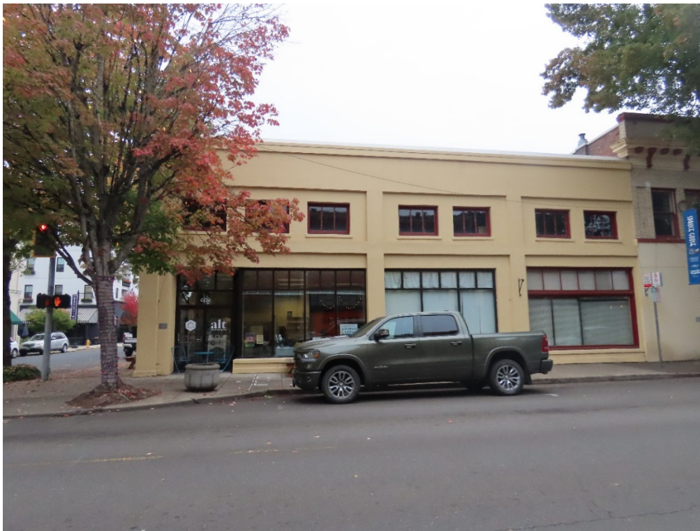
The left two bays of the ground floor have since been infilled with the current street-facing storefront (ARG, October 2022).
