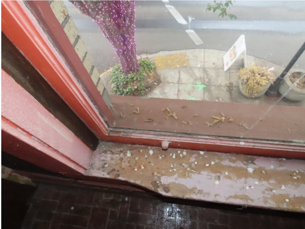
Photo 13. Detail, original second floor window (ARG, October 2022).
