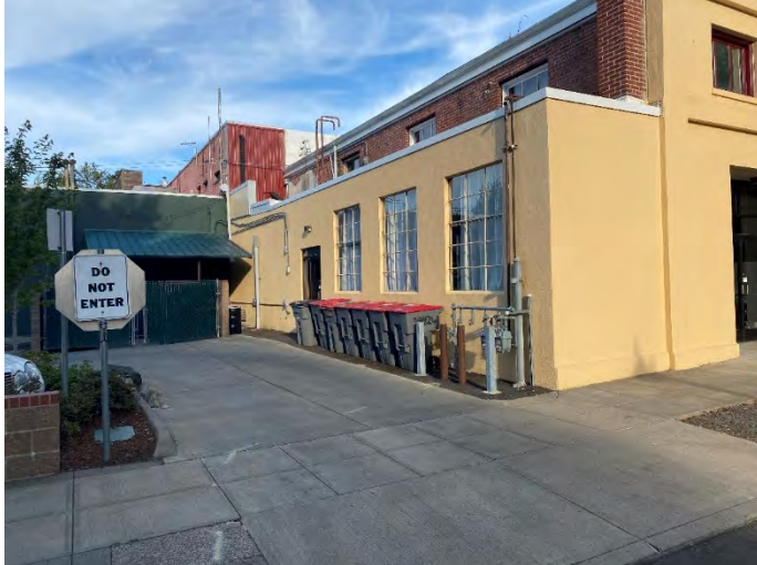
Existing Ford Street Access Location
