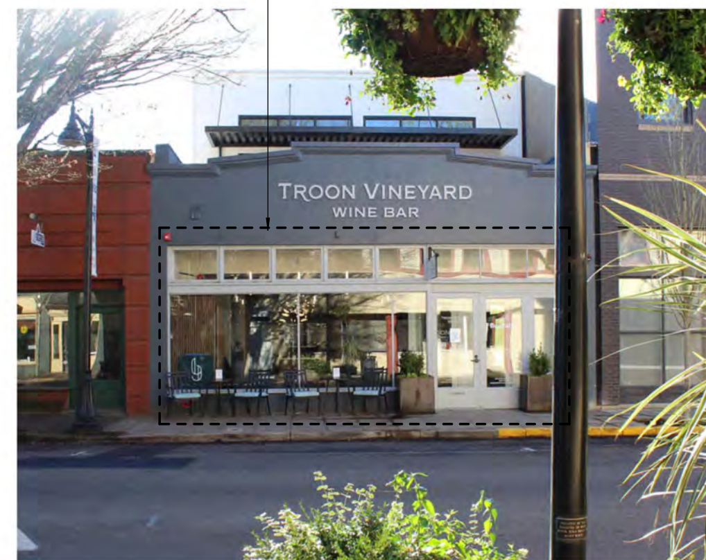
TRADITIONAL WOOD STOREFRONT DETAILING AND TRANSOM
