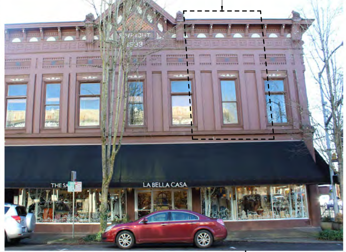
BRICK DETAILING AND RECESSES
