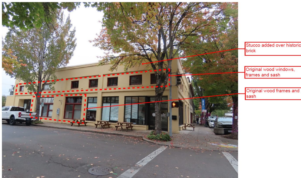
West Elevation facing NE Ford Street, illustrating original features (ARG, October 2022).
