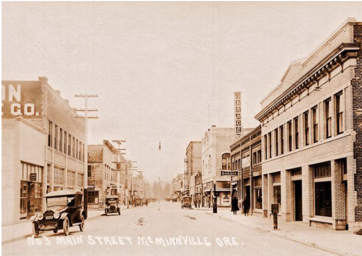
Original Structure, circa 1919
