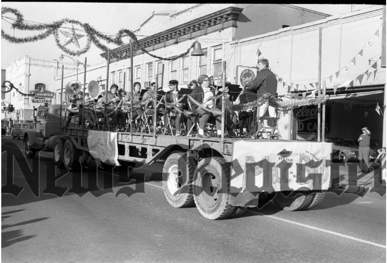
1969 Photo of 619 NE Third Street depicting the automobile bays. (Yamhill County News Register)
