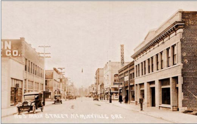
Circa 1919 Photo of 611 NE Third Street depicting two-story brick construction with a decorative parapet and extensive brick corbeling.
