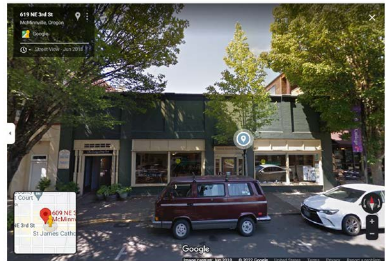
2018, Photo of 619 NE Third Street, the automobile bays have been modified into storefronts, and the brick is painted but the subtle brick decoration is still visible.
