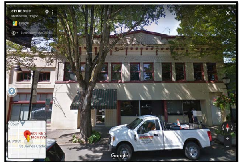
2018, Photo of 611 NE Third Street, shows the modified storefront, but the retention of the original brick, parapet and second floor fenestration pattern.
