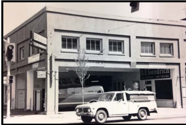
1983 photo of the property shows the modified corner storefront for the gas pumps, the removal of the brick corbeling on the second floor and the stucco veneer that was applied all over., (Historic Resources Survey, City of McMinnville, Yamhill County, Oregon)
