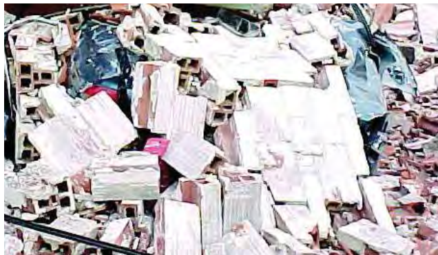
■ Figure 19. URM building damage, 2001 Nisqually, Washington earthquake.
