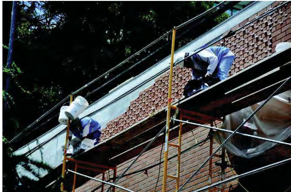
■ Figure 12. Workers installing brick veneer.
