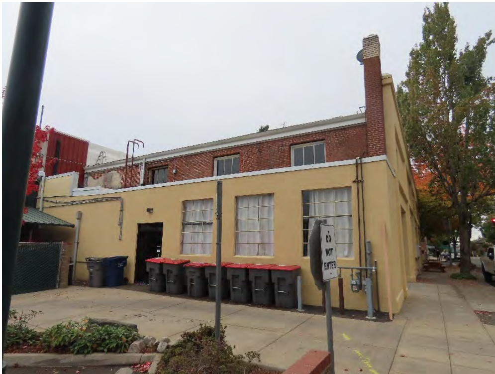
Photo 6. One-story north bay, rear elevation, showing original second floor windows, And steel windows at ground floor (ARG, October 2022).
