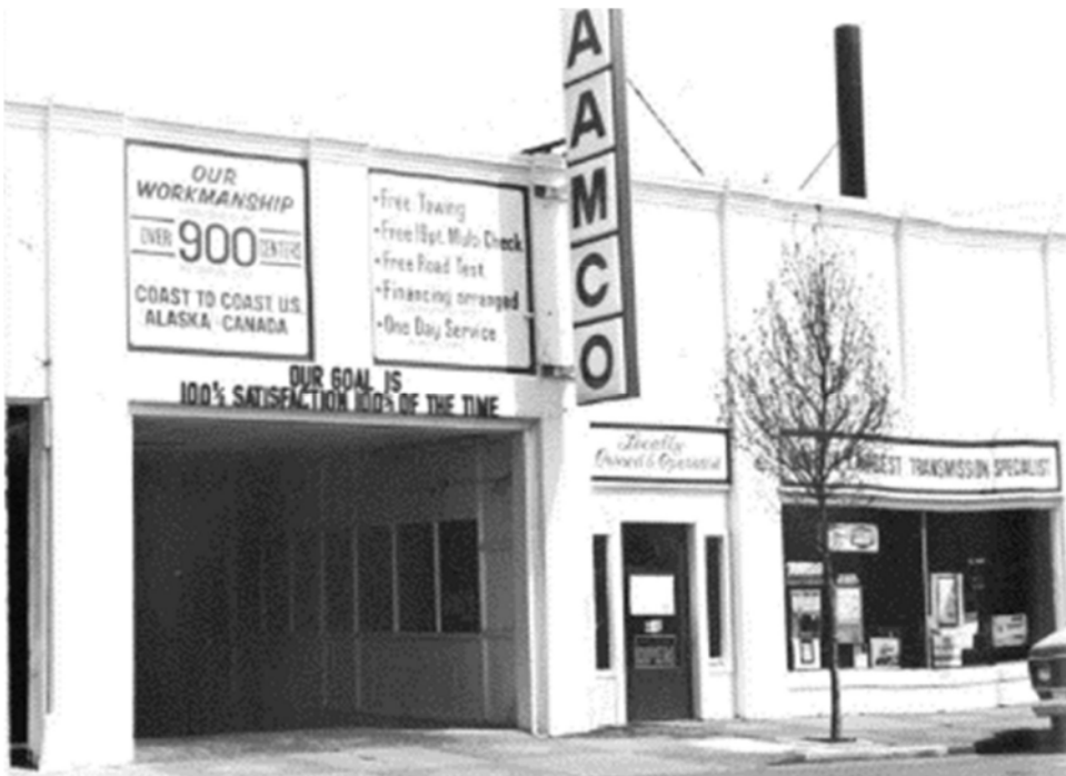
By the time of this 1983 historic survey photograph, the window to the east of the double-wide opening had been converted to an entry and the windows in the two easternmost bays had been replaced with a storefront window spanning both bays (Historic Resources Survey, City of McMinnville, Yamhill County, Oregon).
