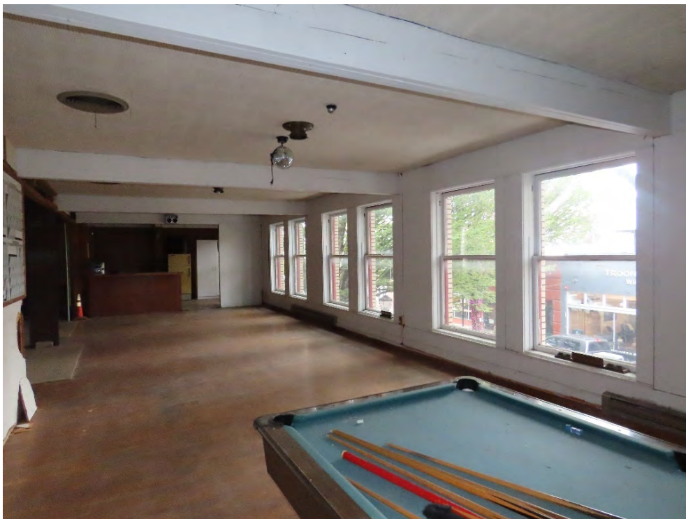
Photo 12. Second floor interior view of original wood windows (ARG, October 2022).
