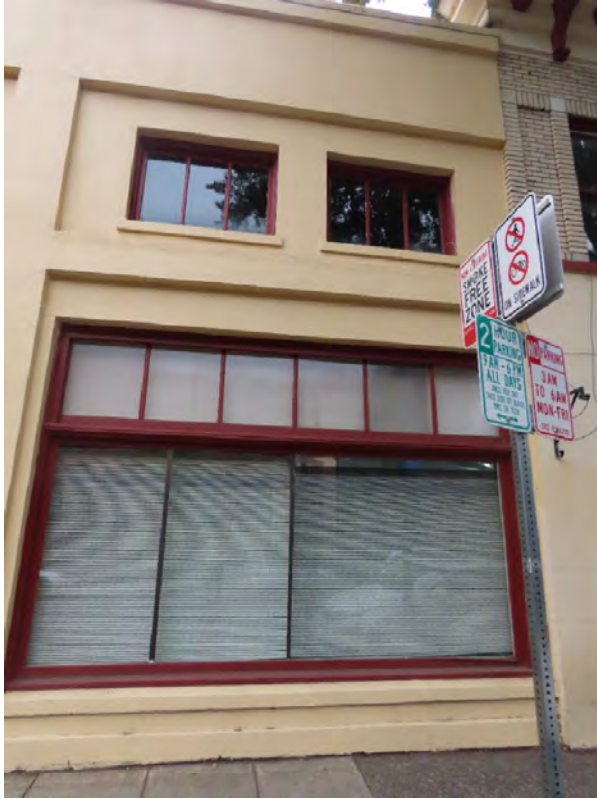
Photo 1. NE 3rd Street elevation: Original wood storefront window and transom, and second-floor windows; storefront has been modified with addition of metal mullions (ARG, October 2022).
