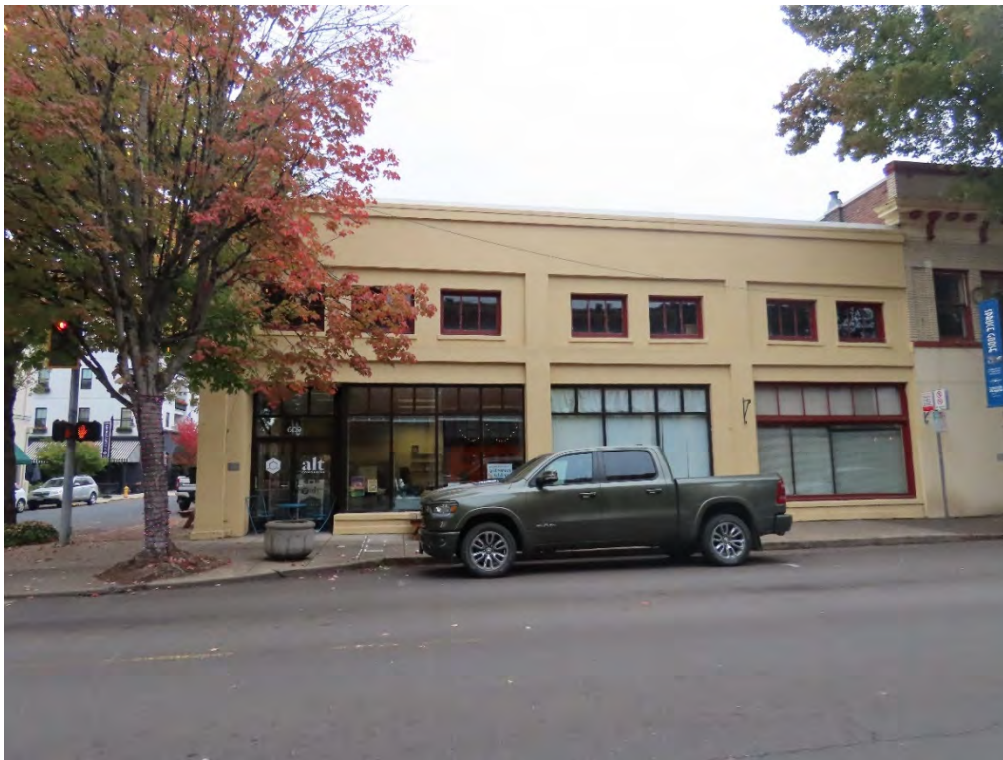
The left two bays of the ground floor have since been infilled with the current street-facing storefront (ARG, October 2022).
