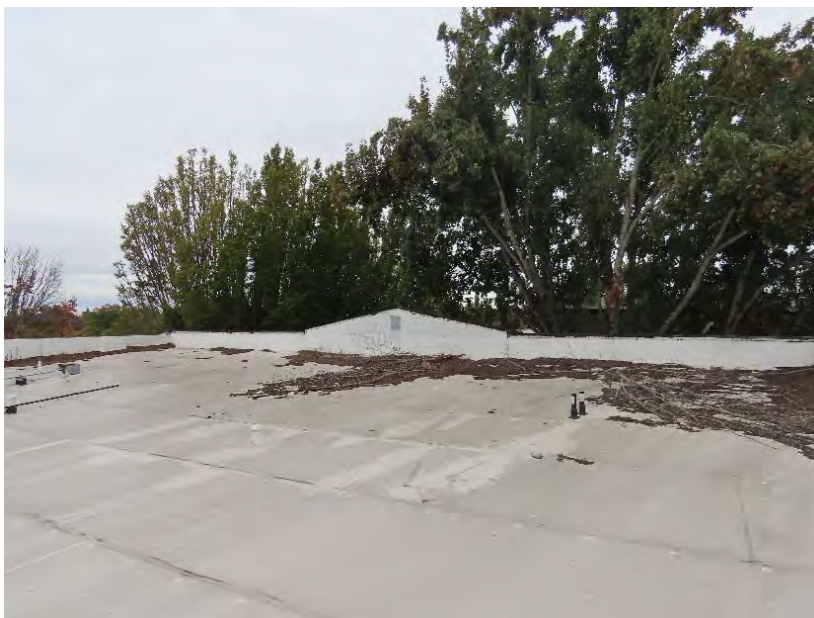
Photo 16. Roof looking south (ARG, October 2022).
