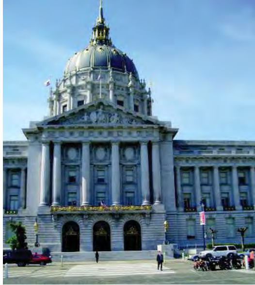
■ Figure 33. The San Francisco City Hall seismic retrofit, which includes seismic isolators. — Robert Reitherman
