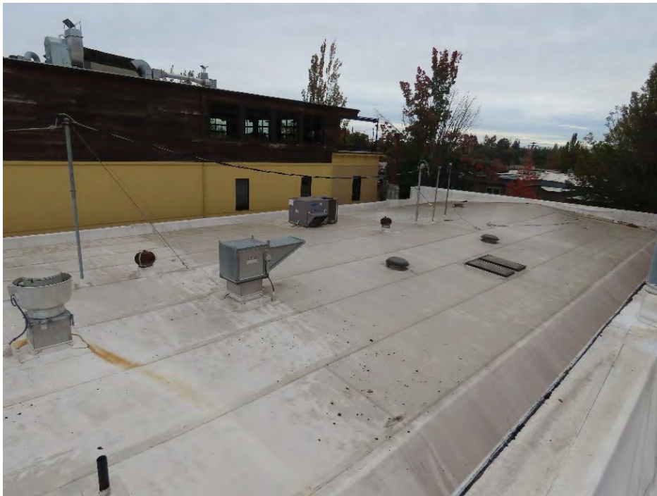
Photo 24. Roof overall view looking south (ARG, October 2022).
