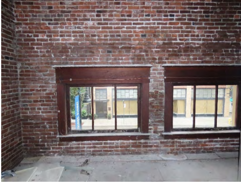
Photo 3. Second floor window, interior view, showing original millwork surrounds (ARG, October 2022).
