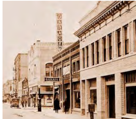
A 1919 photograph looking west along NE 3rd Street showing the original ground floor configuration of 609 NE 3rd Street (Yamhill County News-Register, collection of Michael Hafner).
