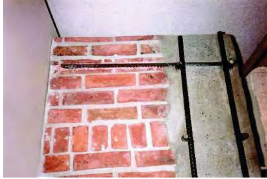
■ Figure 31. California Capitol Retrofit.
