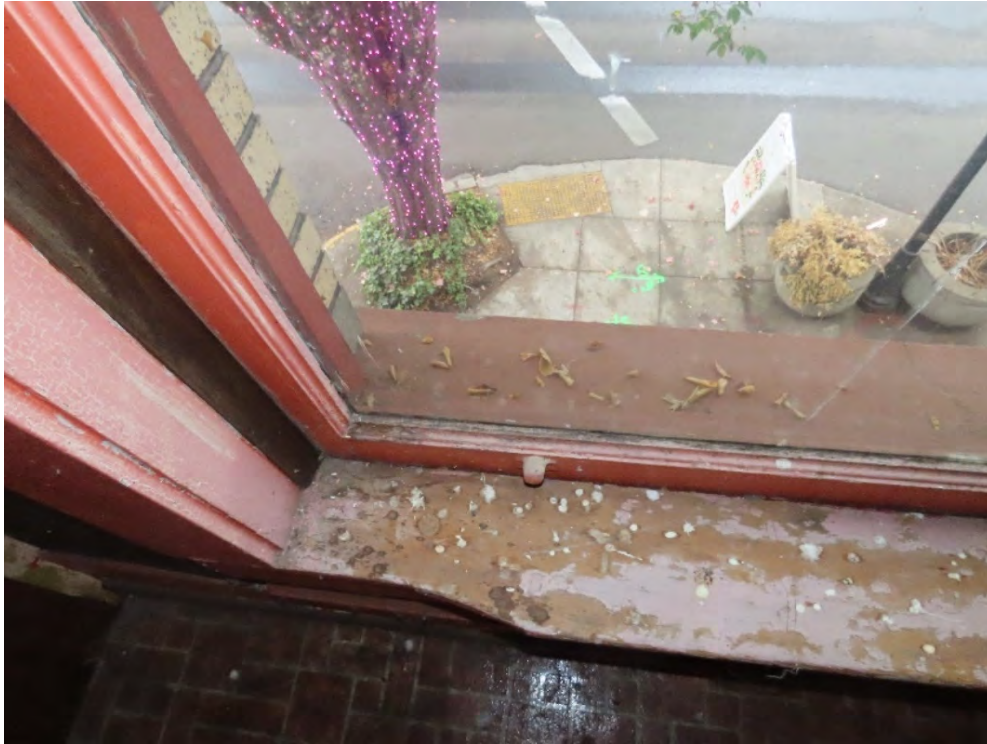
Photo 13. Detail, original second floor window (ARG, October 2022).
