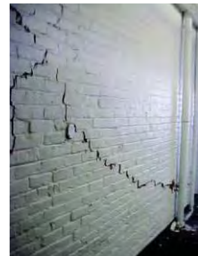
■ Figure 19. URM building damage, 2001 Nisqually, Washington earthquake.
