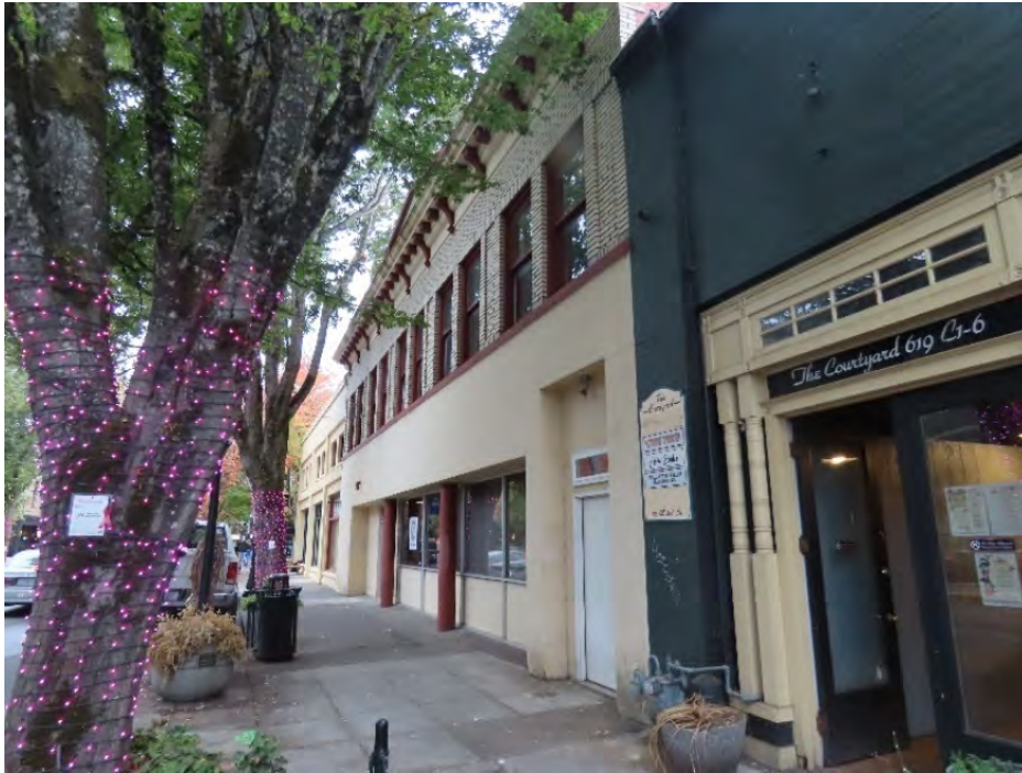
Photo 9. Overall view of south elevation, showing modified ground floor and original second floor (ARG, October 2022).
