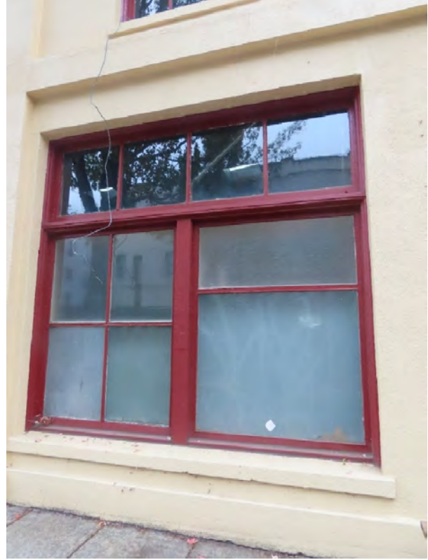
Photo 2. NE Ford Street elevation: Original wood storefront window and transom; mis-matching translucent glass types. Storefront muntins may have been reconfigured (ARG, October 2022).
