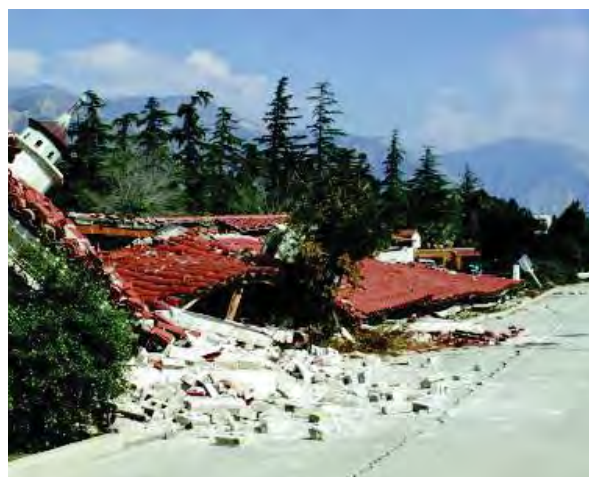
■ Figure 9. Complete collapse of an unreinforced concrete block building, 1971 San Fernando earthquake. —Karl Steinbrugge, NISEE, U.C. Berkeley
