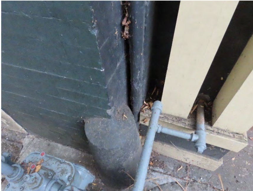
Photo 21. Original brick mould and bollard protector at westernmost opening (ARG, October 2022).
