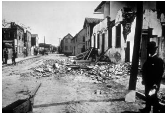
■ Figure 13. Debris resulting from the 1886 Charleston, South Carolina earthquake. —NISEE, U.C. Berkeley
