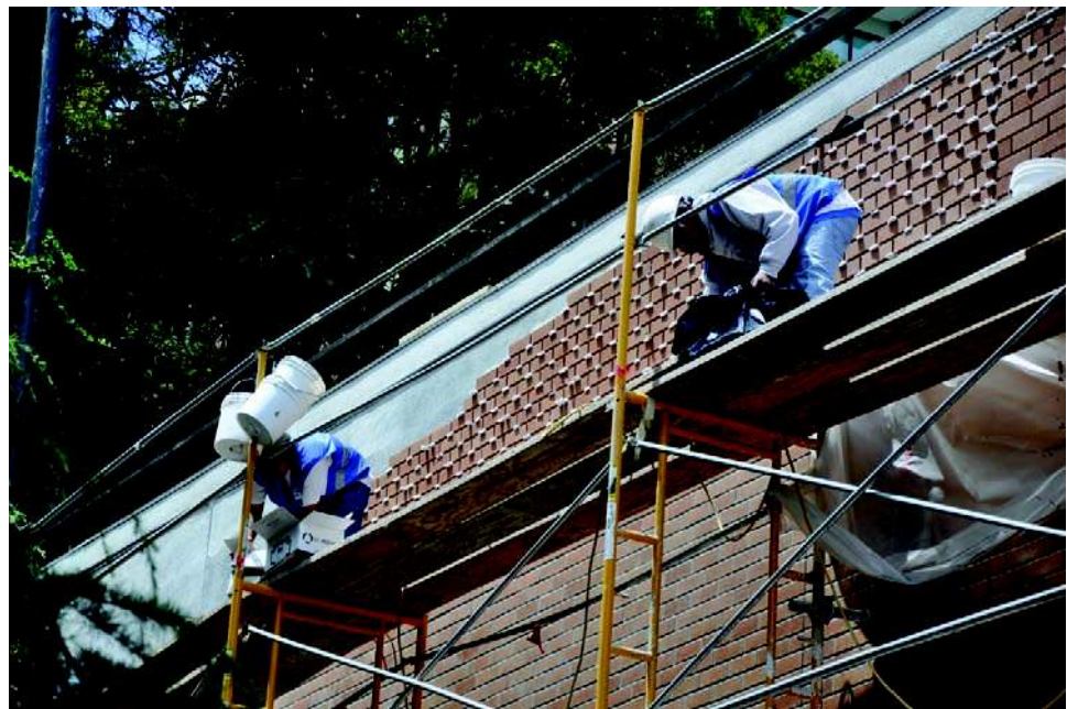
■ Figure 12. Workers installing brick veneer.
