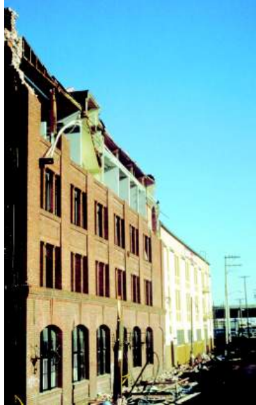
■ Figure 18. Upper story wall collapse, with resulting fatalities.
