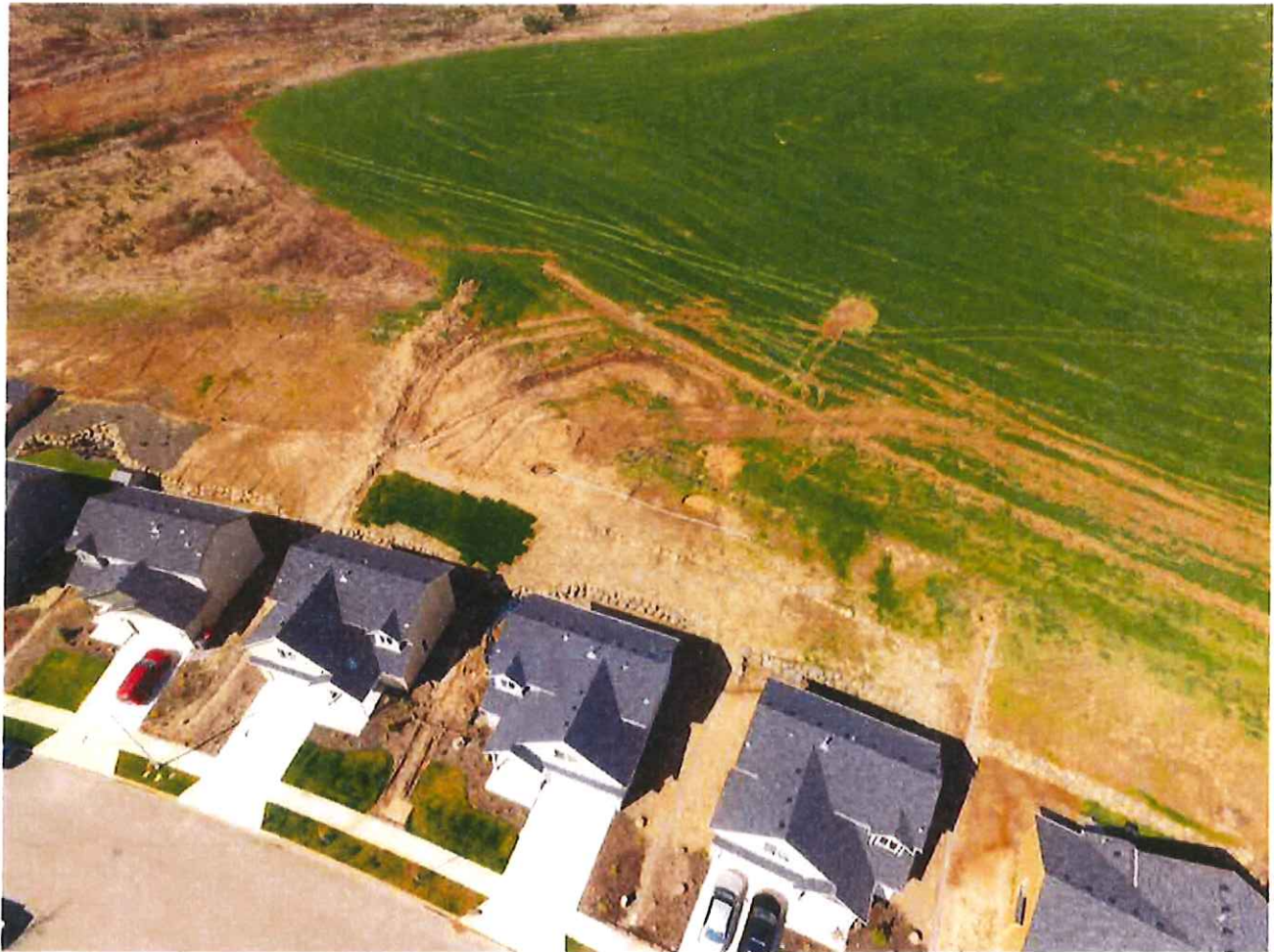
Existing, Recently Active Landslide – View to the North March 17, 2016
