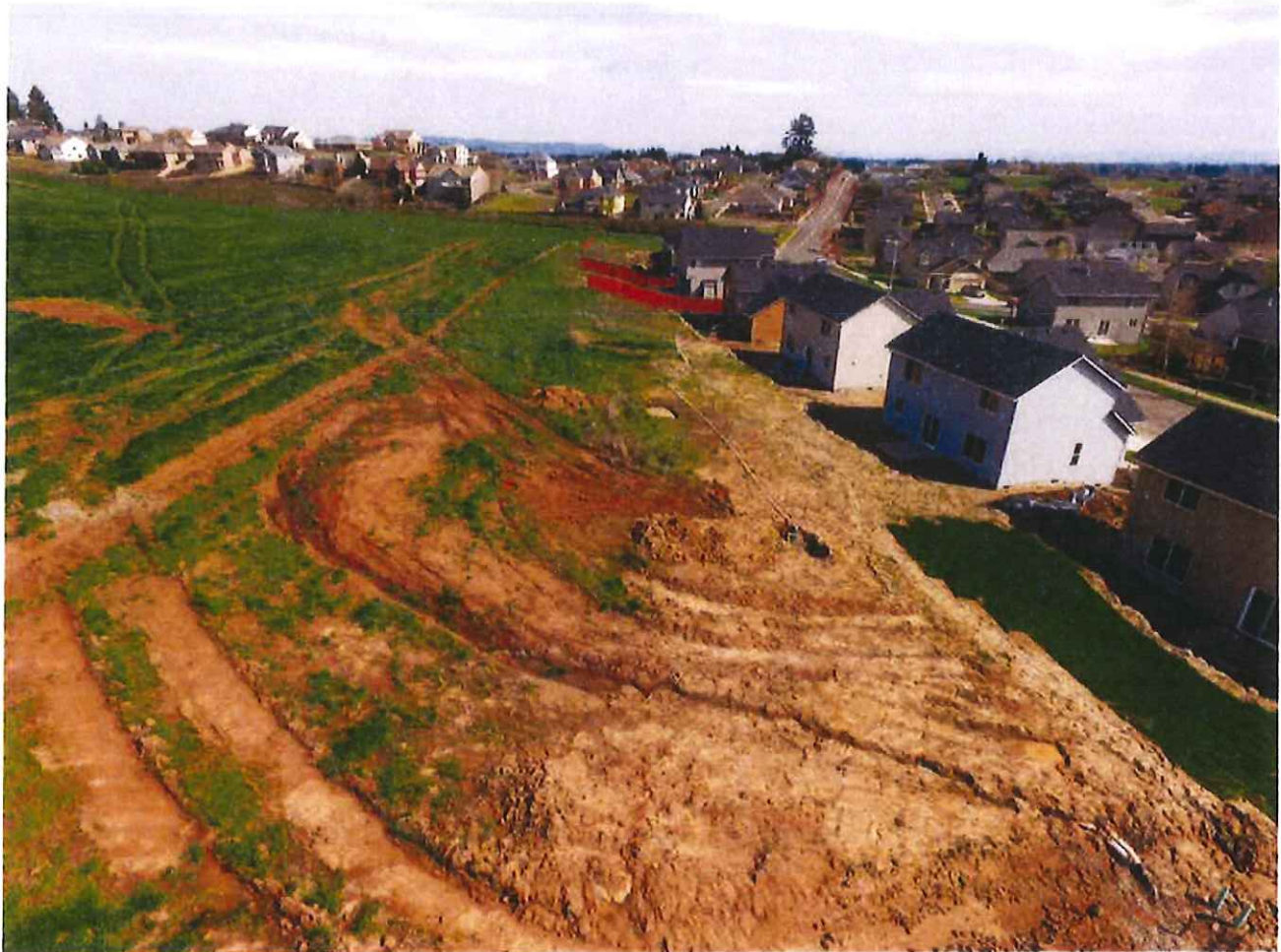
Existing, Recently Active Landslide – View to the East March 17, 2016
