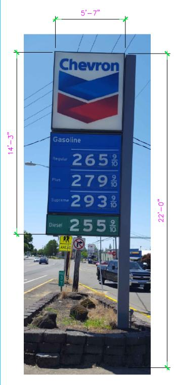
Sign post shortened, and sign cabinet lowered to 20' sign height to meet city ordinance. Lower Diesel cabinet removed, face of existing price cabinet replaced with new LED face to achieve the maximum vision clearance while meeting new Chevron standards.
