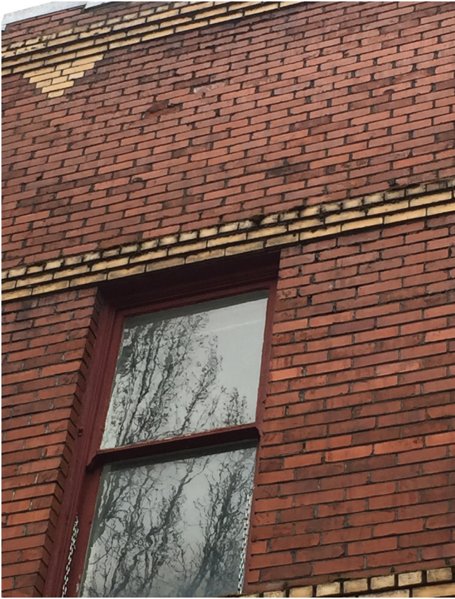
SPALLING BRICK AT WEST FACADE
