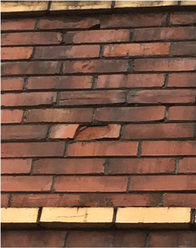
SPALLING BRICK AT WEST FACADE
