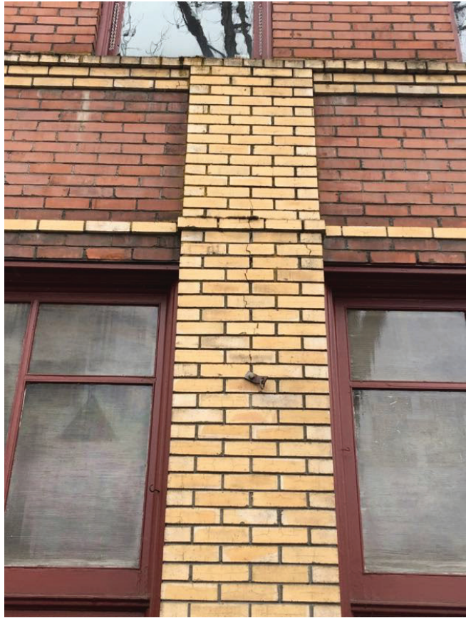
CRACKING IN BUFF-COLORED BRICK AT COLUMNS AND RUSTING OF STEEL LINTELS AT NORTH AND WEST FACADES
