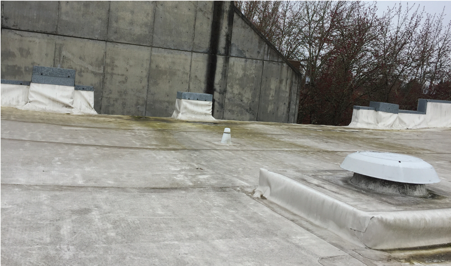
ROOF, LOOKING SOUTH TOWARD CHIMNEYS AT ALLEY
