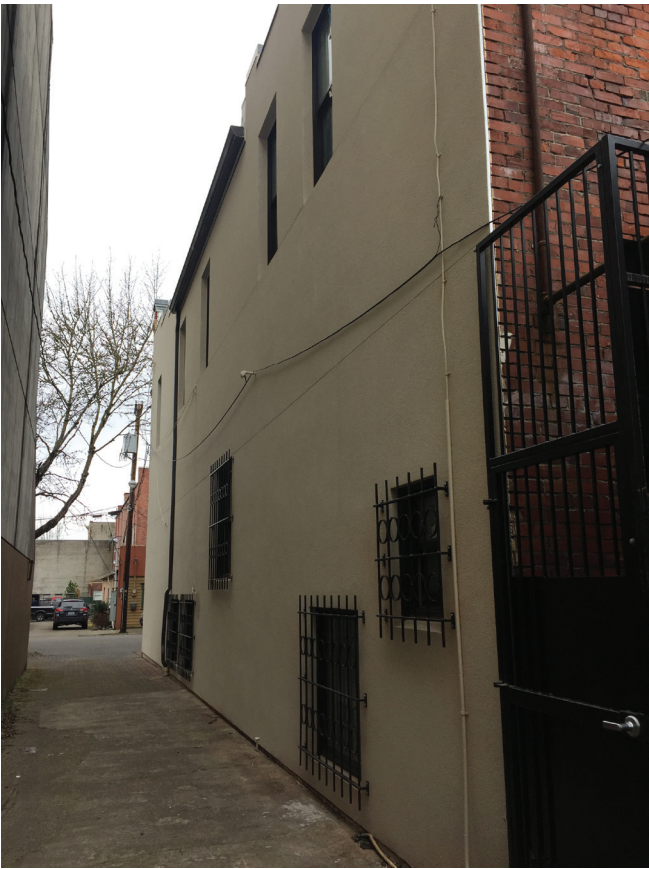
SOUTH FACADE (ALLEY) AS SEEN FROM SOUTHEAST
