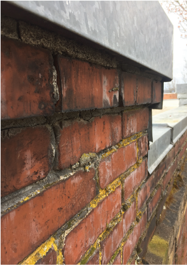
DETERIORATED MORTAR JOINTS AND ORGANIC GROWTH
