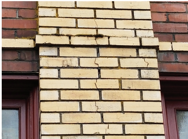
CRACKING IN BUFF-COLORED BRICK AT COLUMNS AND RUSTING OF STEEL LINTELS AT NORTH AND WEST FACADES
