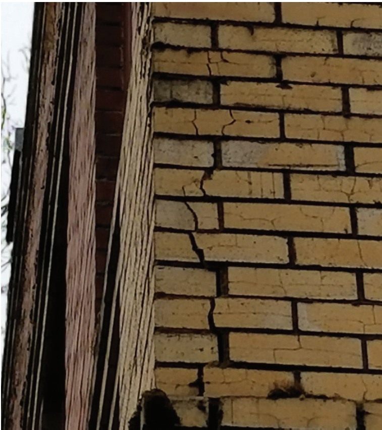
CRACKING IN BUFF-COLORED BRICK AT COLUMNS AND RUSTING OF STEEL LINTELS AT NORTH AND WEST FACADES
