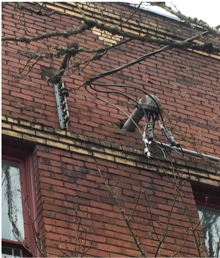
ELECTRICAL SERVICE PENETRATING BRICK
