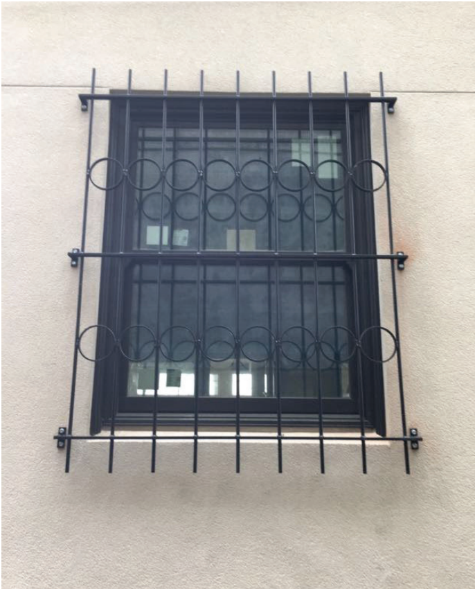
TYPICAL WINDOW AT SOUTH FACADE
