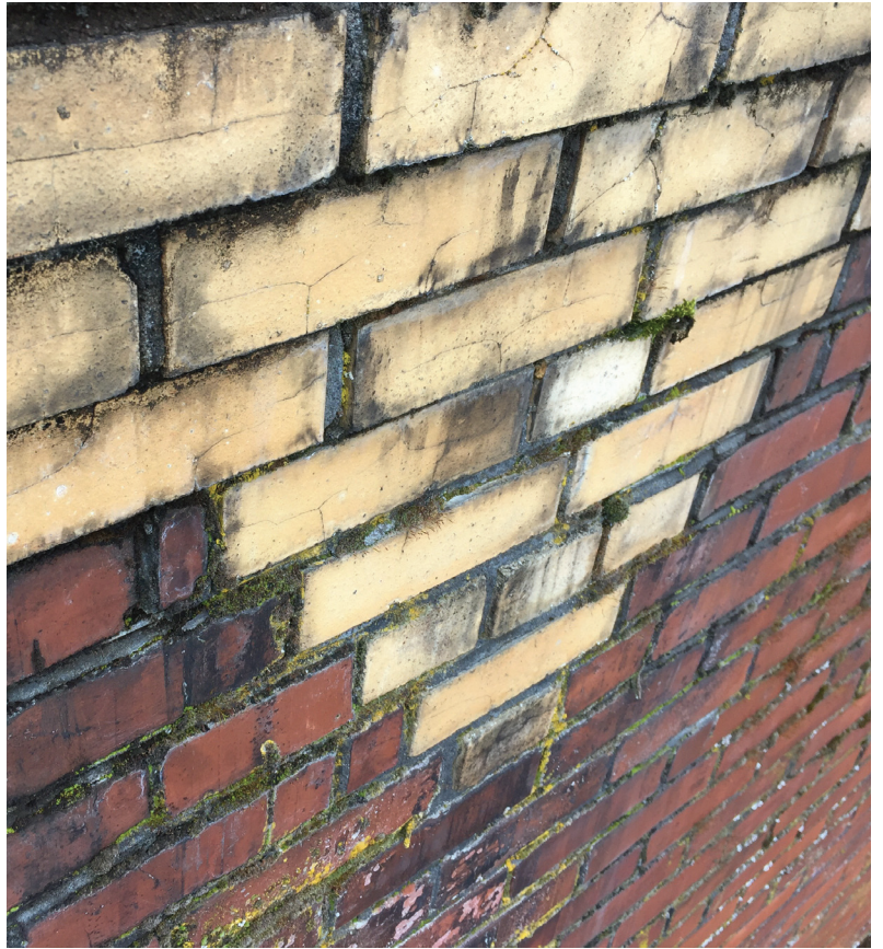
DETERIORATED MORTAR JOINTS AND ORGANIC GROWTH
