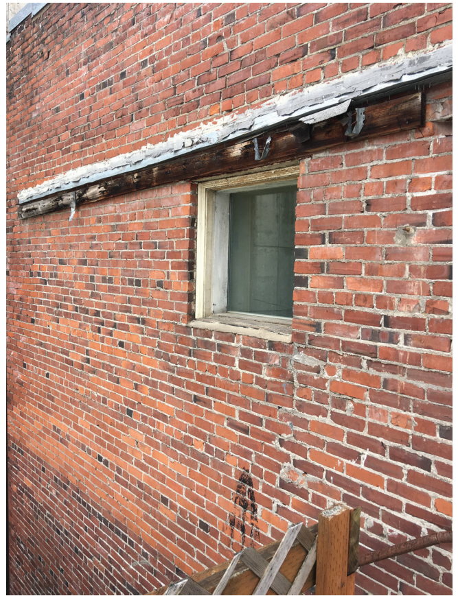
ROOF DECK LEDGER AT EAST FACADE
