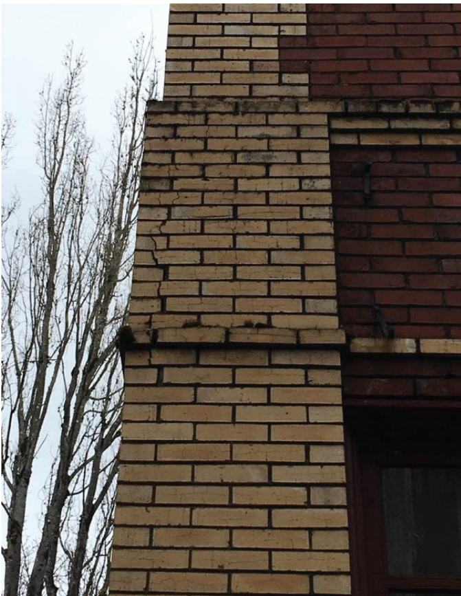
CRACKING AT BUFF-COLORED BRICK
