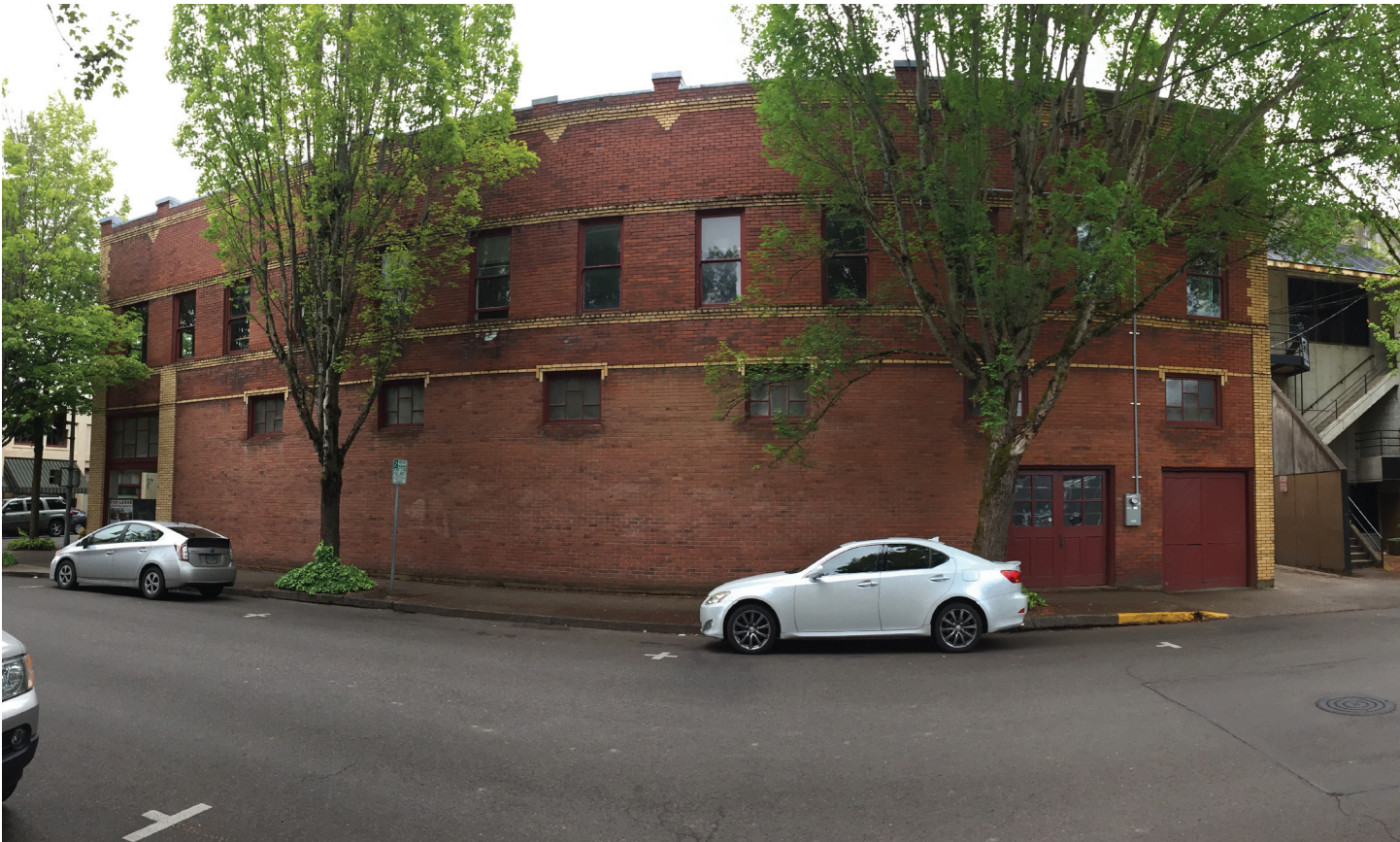
WEST FACADE (FORD STREET)
