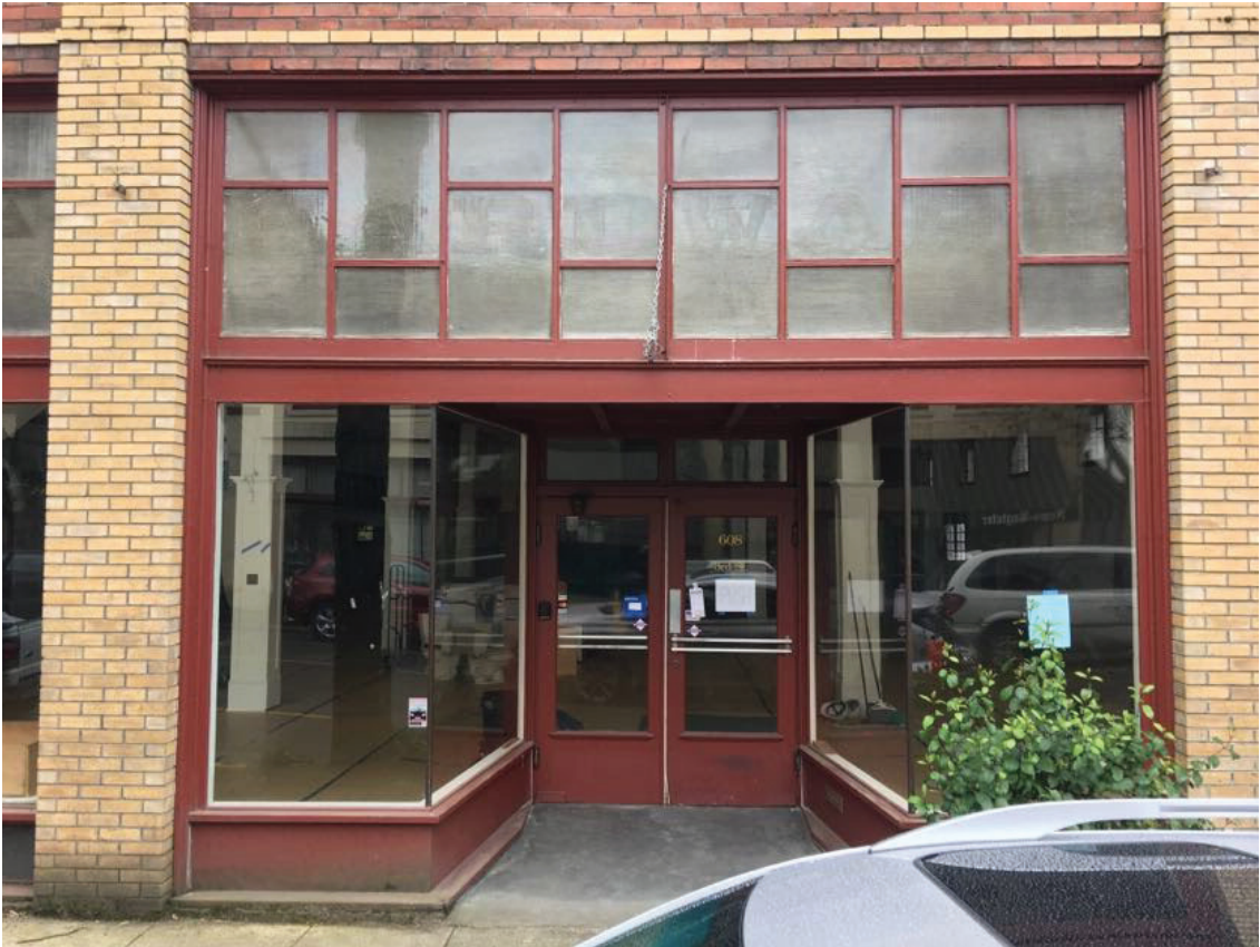
MAIN FLOOR ENTRANCE AT NORTH FACADE
