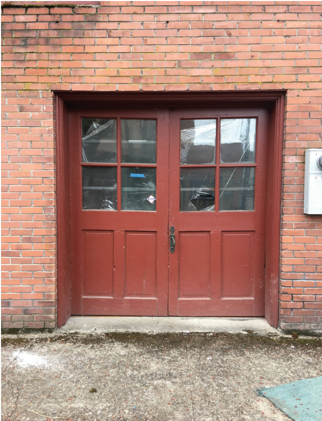
DOUBLE DOOR ENTRANCE
