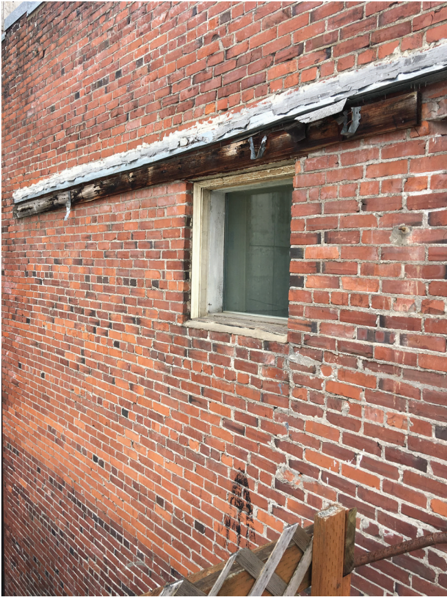
ROOF DECK LEDGER AT EAST FACADE
