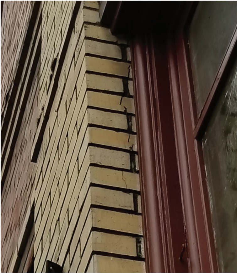
CRACKING IN BUFF-COLORED BRICK AT COLUMNS AND RUSTING OF STEEL LINTELS AT NORTH AND WEST FACADES
