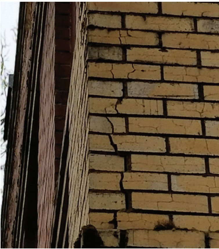
CRACKING IN BUFF-COLORED BRICK AT COLUMNS AND RUSTING OF STEEL LINTELS AT NORTH AND WEST FACADES
