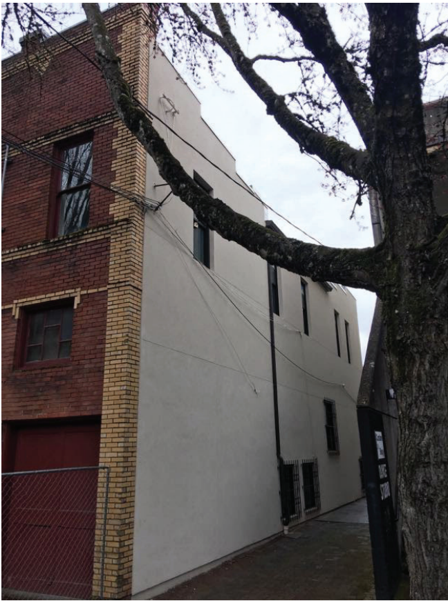
SOUTH FACADE (ALLEY) AS SEEN FROM FORD STREET
