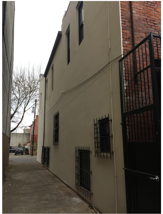
SOUTH FACADE (ALLEY) AS SEEN FROM SOUTHEAST
