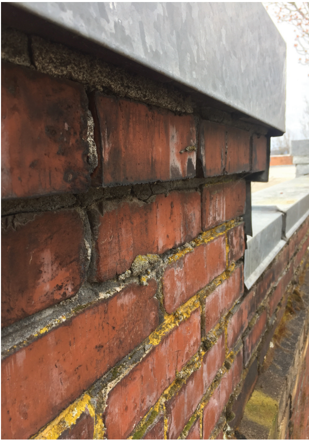
DETERIORATED MORTAR JOINTS AND ORGANIC GROWTH
