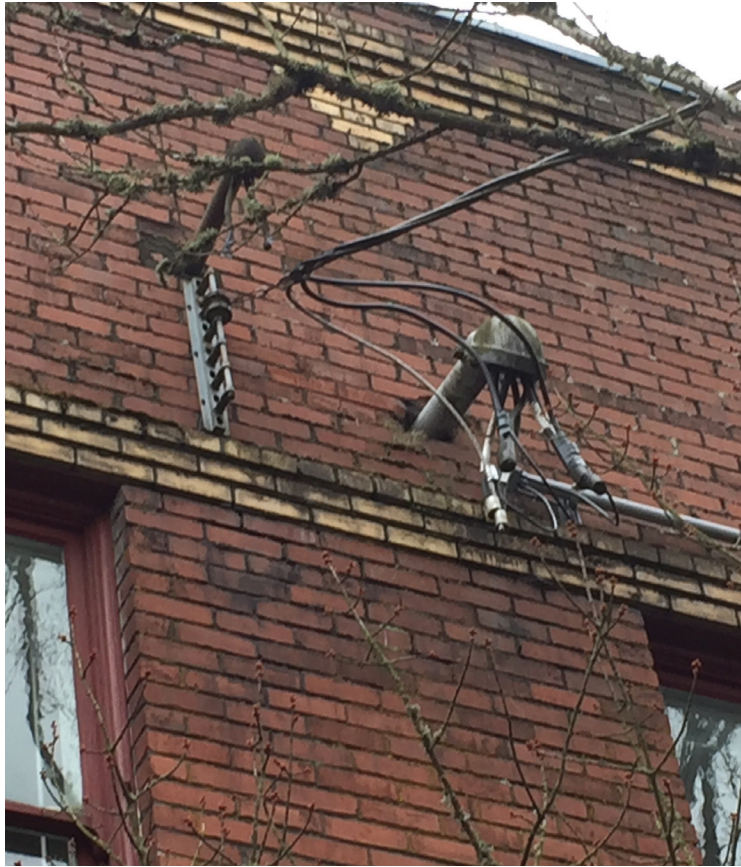
ELECTRICAL SERVICE PENETRATING BRICK
