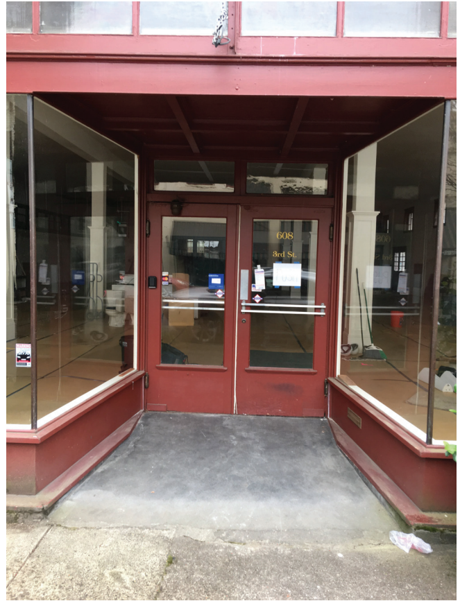
MAIN FLOOR ENTRANCE AT NORTH FACADE
