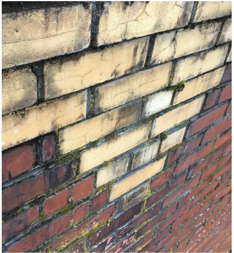
DETERIORATED MORTAR JOINTS AND ORGANIC GROWTH
