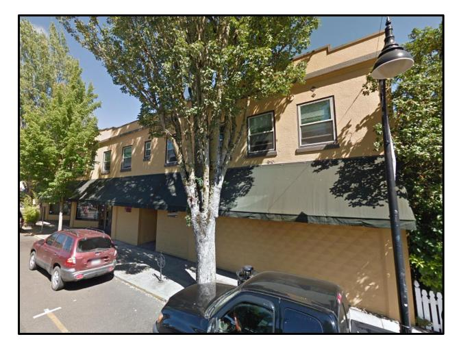
The applicant is proposing to remove an existing concrete block wall on the two easternmost bays of the Third Street ground floor façade and construct in its place two sets of recessed storefront window systems and entries. More specifically, the applicant is proposing to complete the following work on the building:
