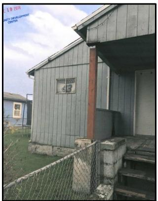
The statement of historical significance also describes the structure as follows: "The north and west façade is resided in plywood while the east and portions of the north façade have asbestos shingle sidsing [sic] over the original horizontal siding." The applicant has stated that the "original horizontal siding and plywood have been replaced with T-1-11 siding". Photos of the absence of these features are provided below:
