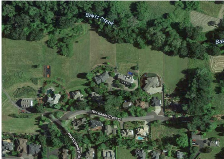
Crestbrook 1 st Addition – fill to accommodate housing, cul-de-sac
