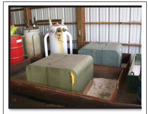
Damaged Transformers in Containment
