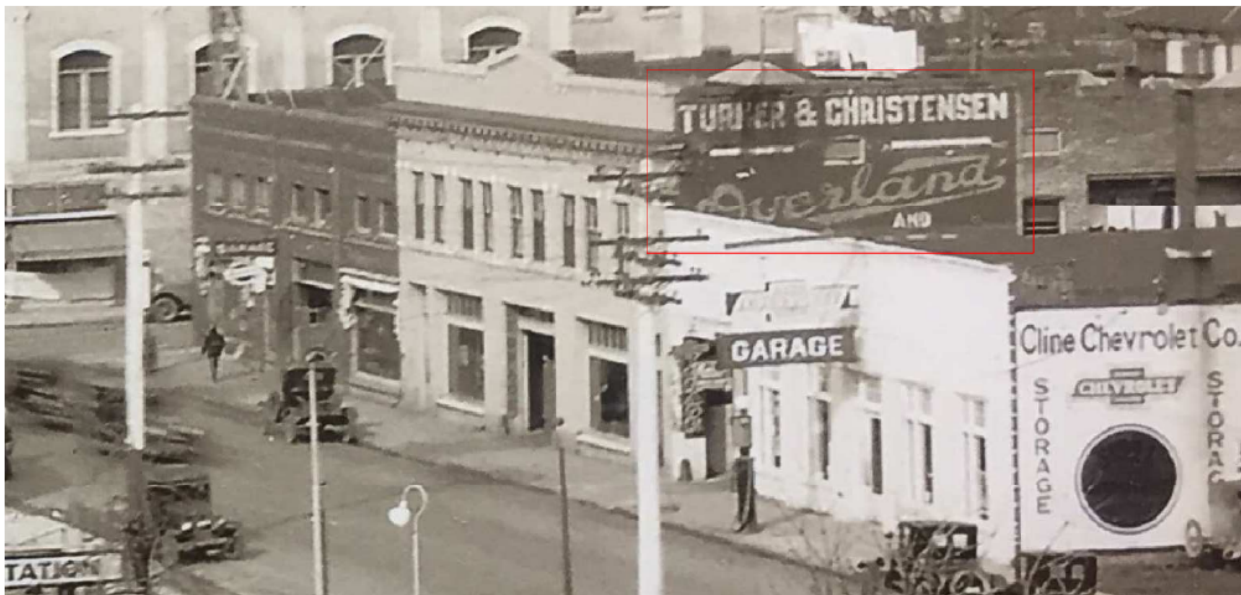
Figure 11 609, 611, and 619 NE 3rd Street McMinnville, 1927
