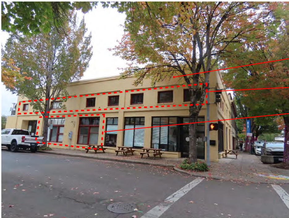
West Elevation facing NE Ford Street, illustrating original features (ARG, October 2022).
