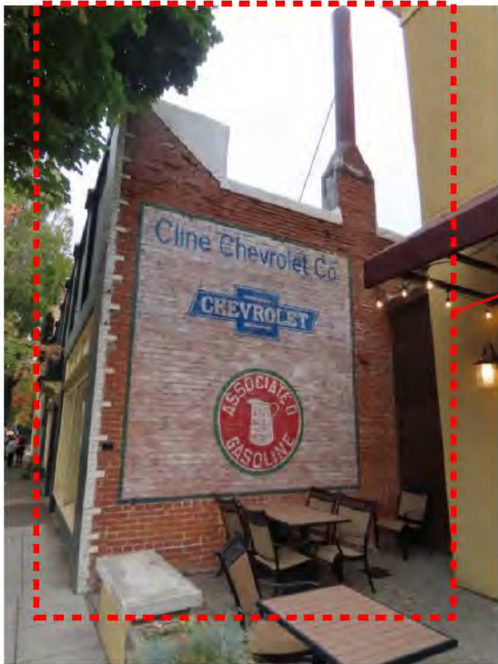
619 NE 3rd Street, Southwest corner, showing restored signage at east elevation (ARG, October 2022).
