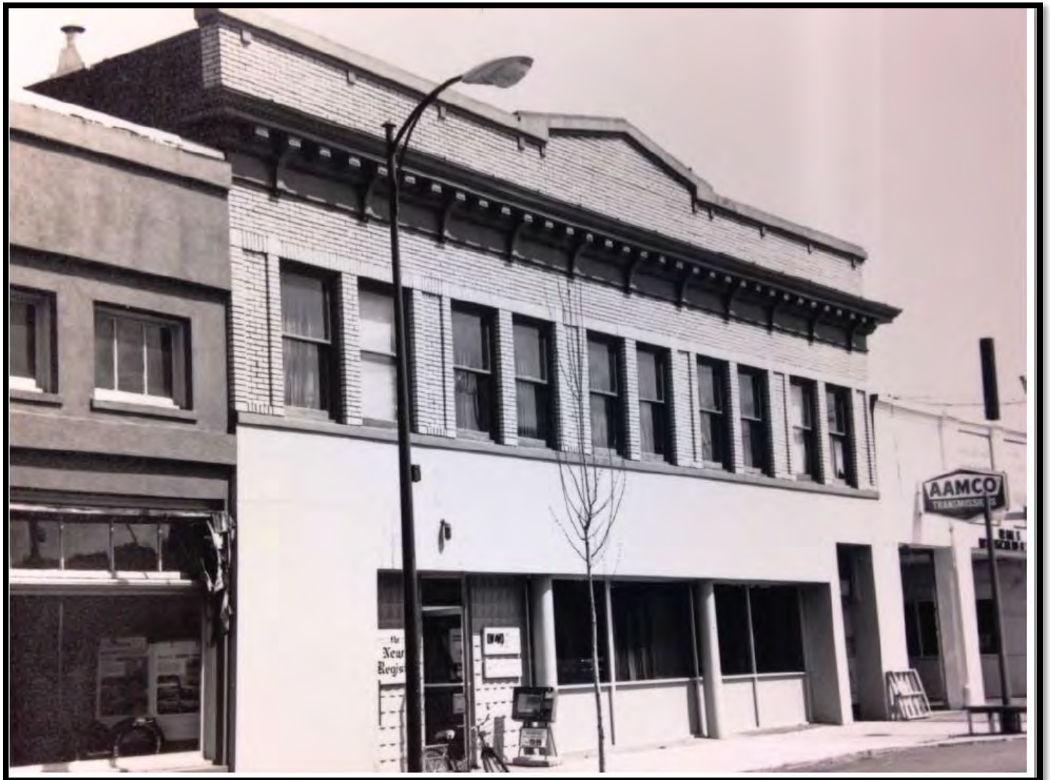
1983 photo of the property shows the modified ground floor storefronts, but with the retention of the original brickwork, parapet and second floor fenestration pattern, (Historic Resources Survey, City of McMinnville, Yamhill County, Oregon)
