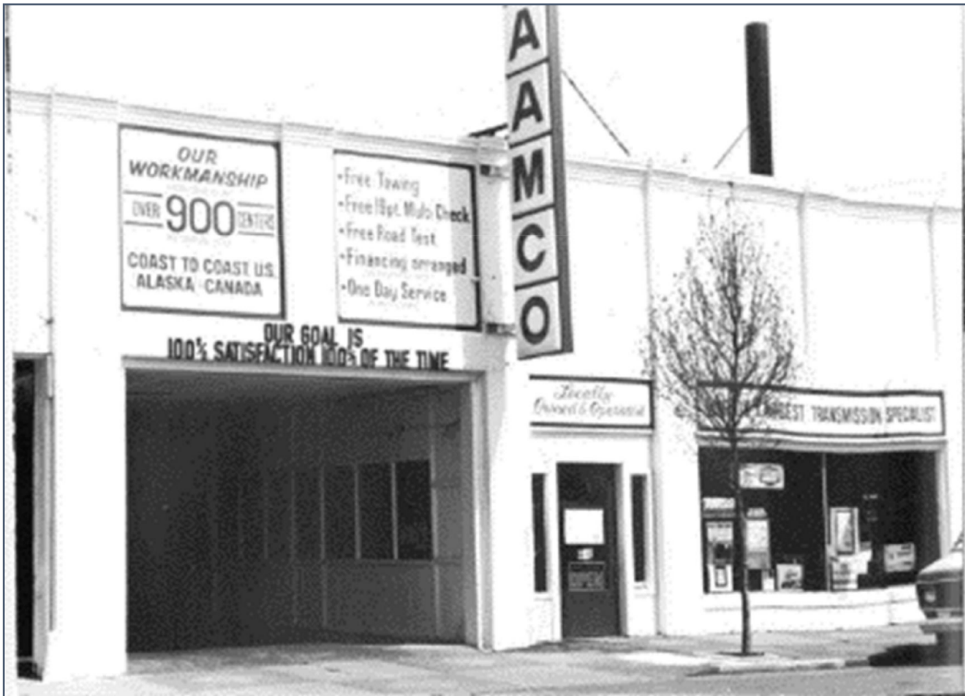
1983 photo of the property shows the modified automobile bays and decorative brick work. (Historic Resources Survey, City of McMinnville, Yamhill County, Oregon)
