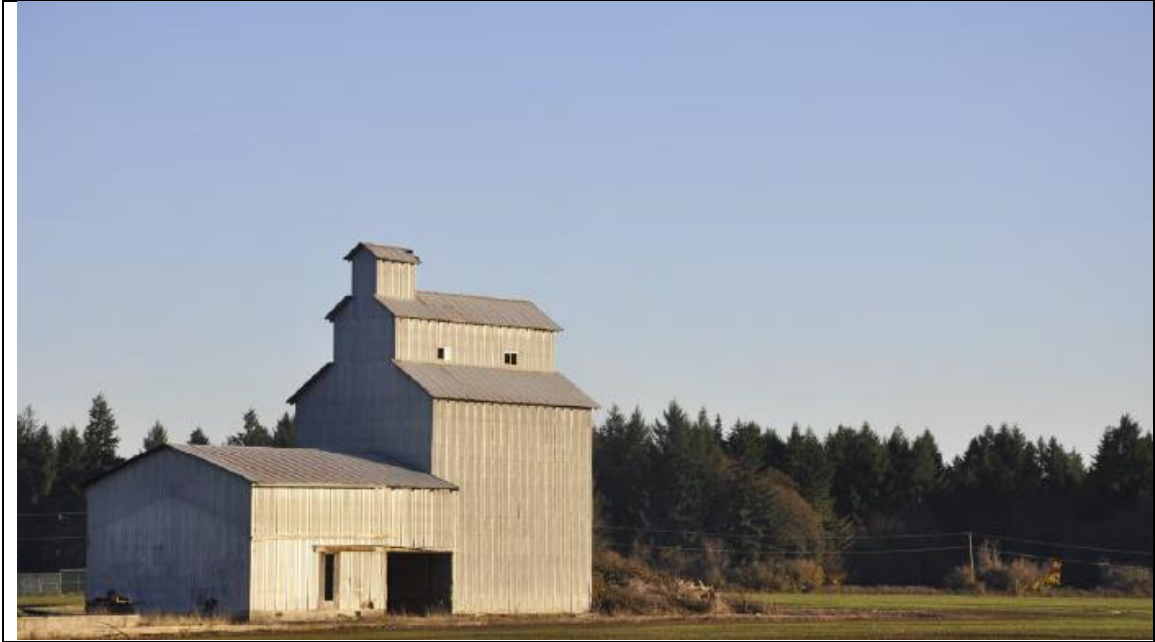
Reference Designs in 3ML Area for Design Treatments for Large Format Retail Stores (from Evergreen Campus Concept Graphics)
