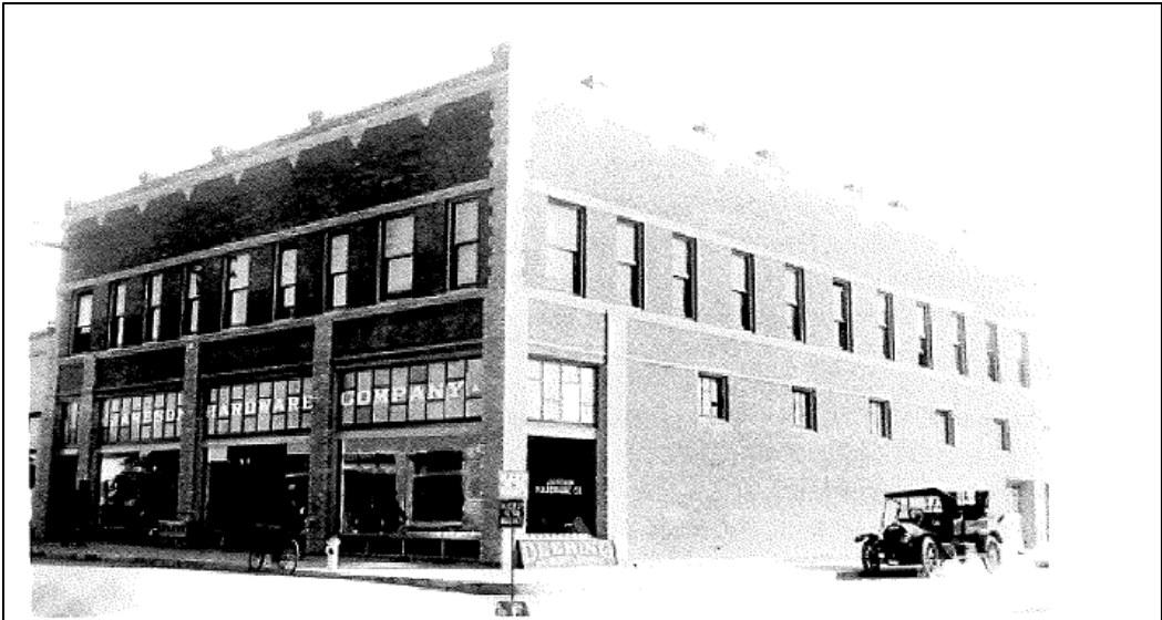
Figure 15: North and West elevations of 608 E. Third St.ca 1918
