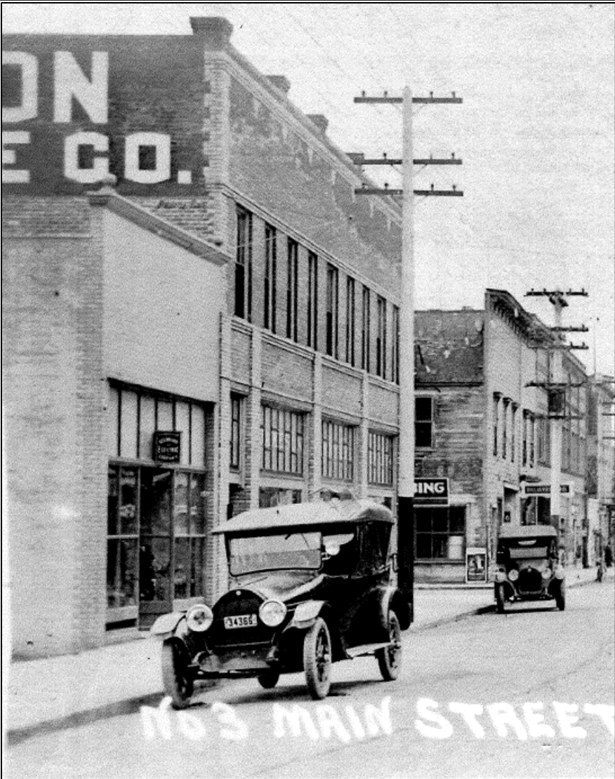
Figure 16: North facades of 618 and 608 3rd Street "No 3 Main Street" Undated, Thought to be ca 1918-1920
