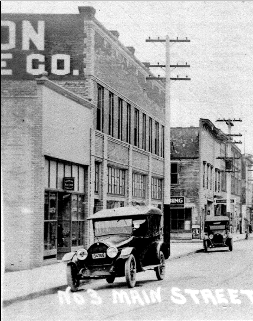
Figure 16: North facades of 618 and 608 3rd Street "No 3 Main Street" Undated, Thought to be ca 1918-1920
