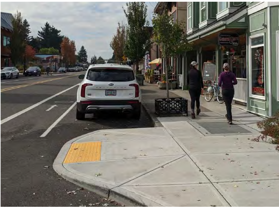
New curb ramps (Historic Columbia River Hwy - Troutdale, OR)
