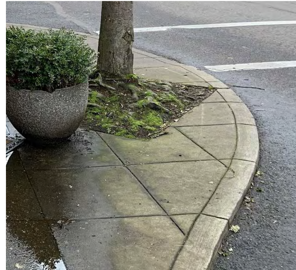
6" Concrete Curb (Existing)
