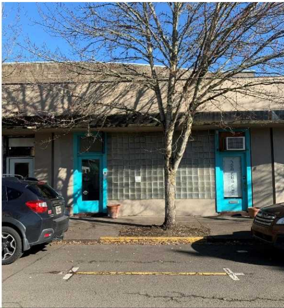
Example of yellow paint between parallel parking stalls on Evans Street
