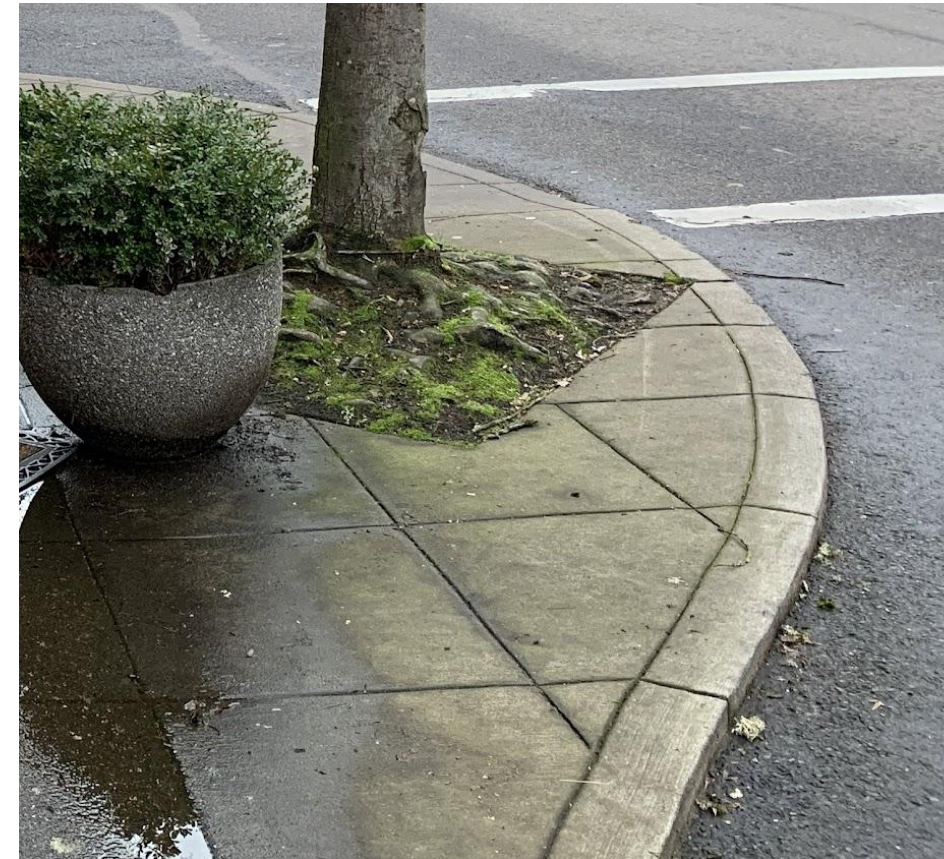
6" Concrete Curb (Existing)
