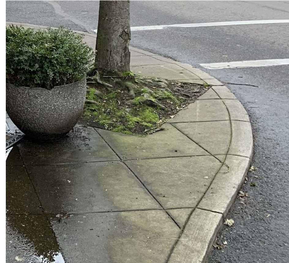
6" Concrete Curb (Existing)
