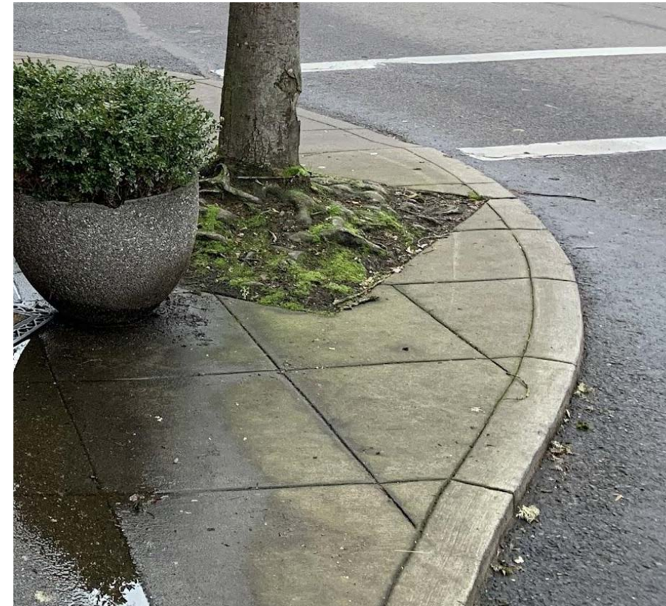
6" Concrete Curb (Existing)
