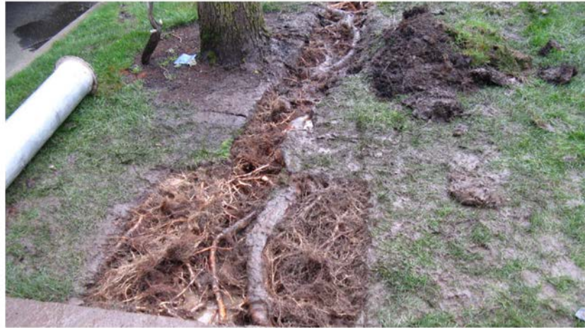
Impractical to demolish street, dig trenches, and reconstruct around large root systems
