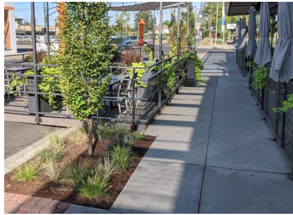
New sidewalks and planter wells (Downtown Walla Walla, WA)
