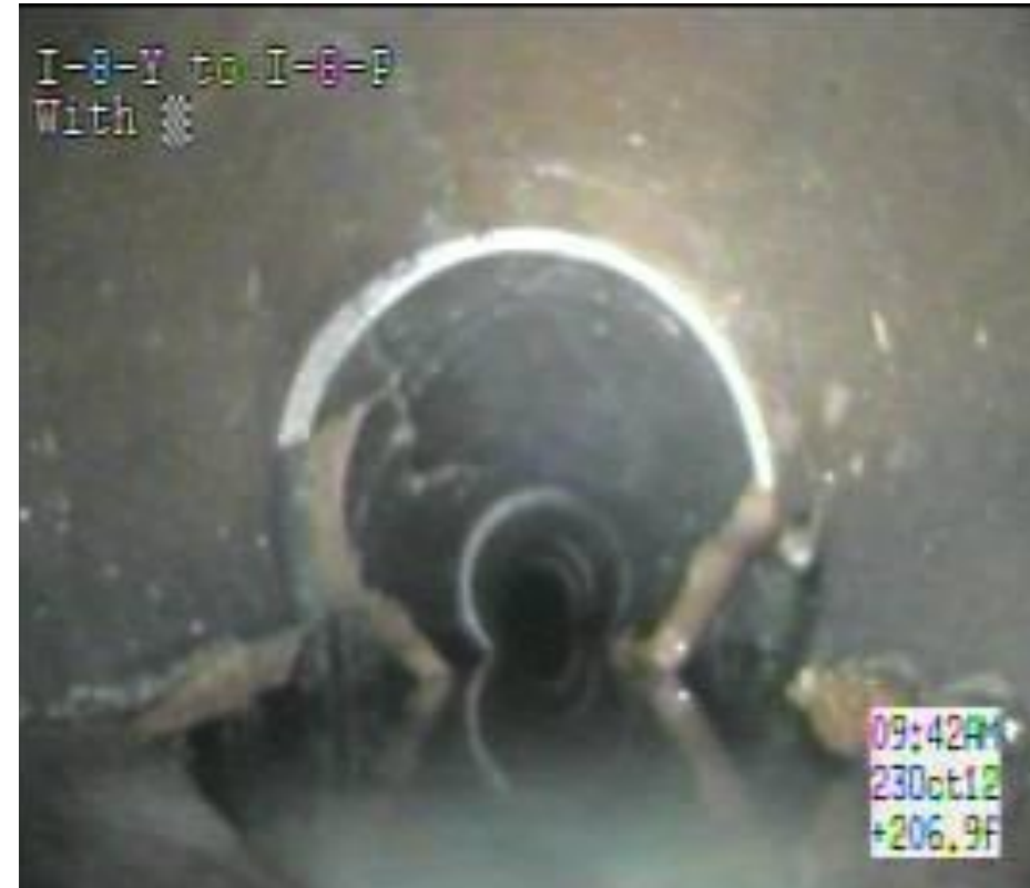
Storm pipe at NE 3rd and Davis
