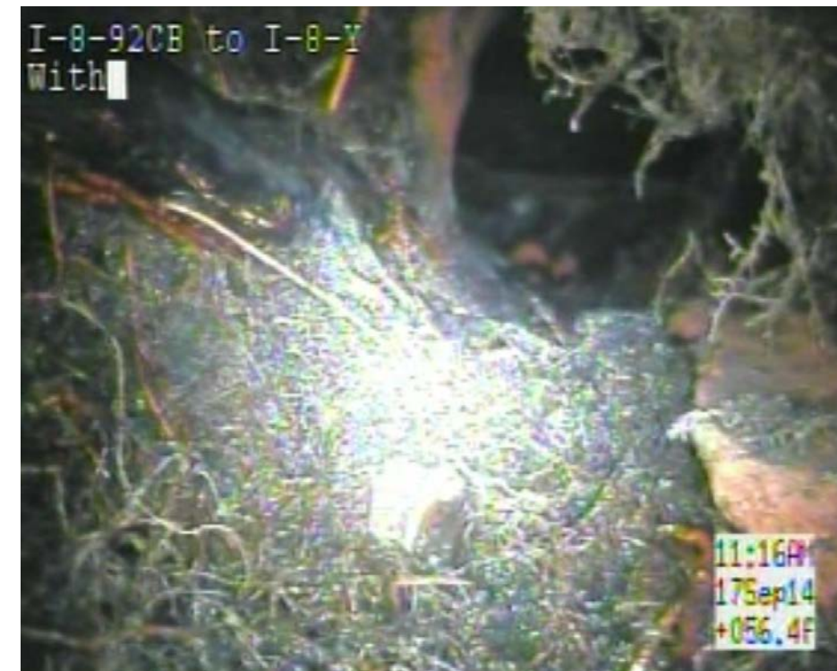
Storm pipe at NE 3rd and Davis
