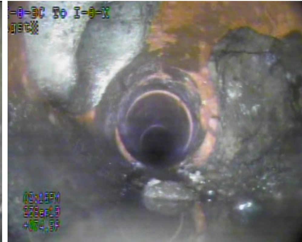
Storm pipe at NE Ford between 3rd and 4th
